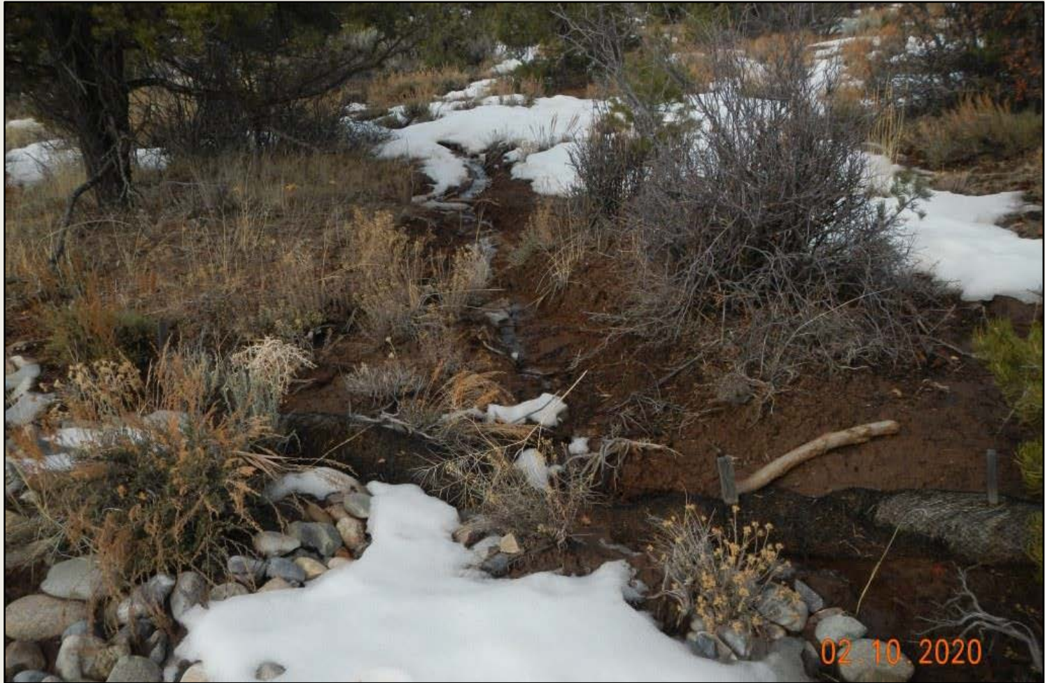
Photo 3. View of area at the northeastern edge of project area where snow melt is forming an erosional channel flowing off of the project area where stormwater controls are not sufficient to de-energize and filter flows.
