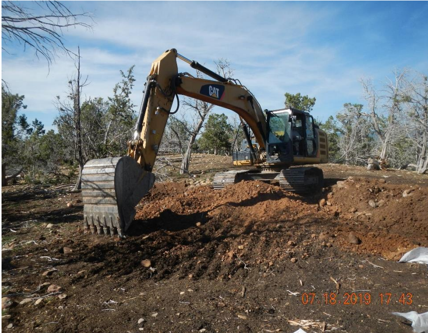
Excavated area backfilled with clean fill.
