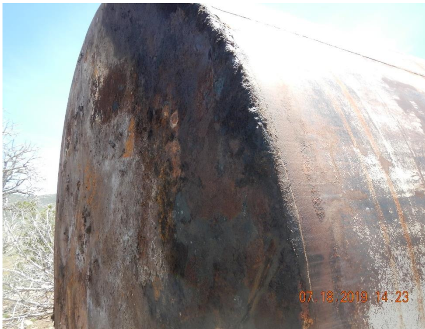
Corrosion along bottom seam of AST.
