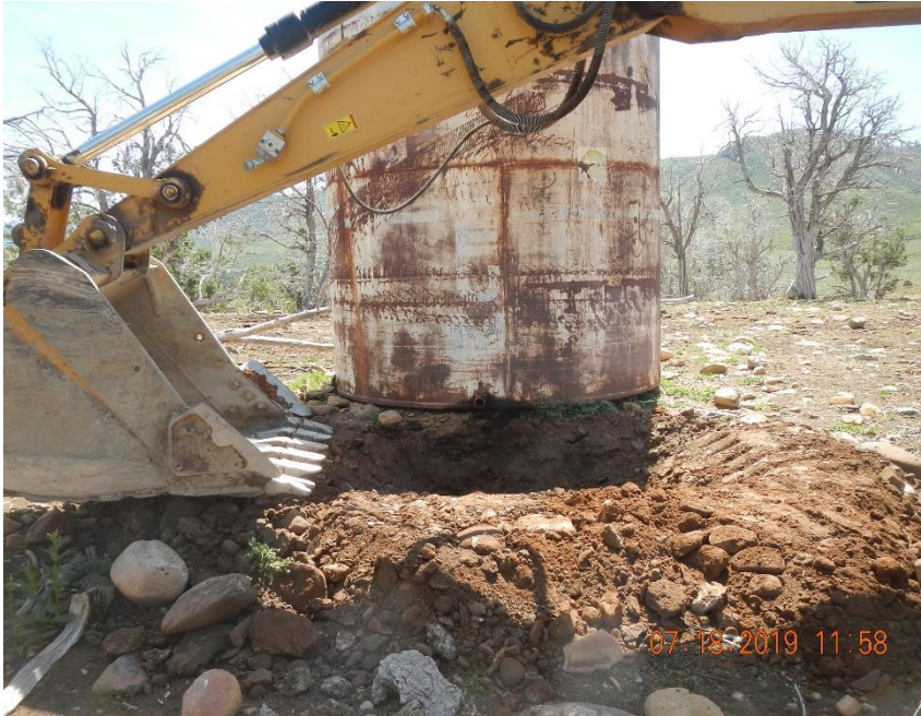
Track hoe excavating containment area.
