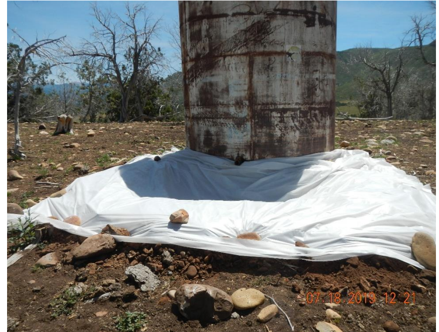
Containment area lined with plastic sheeting.
