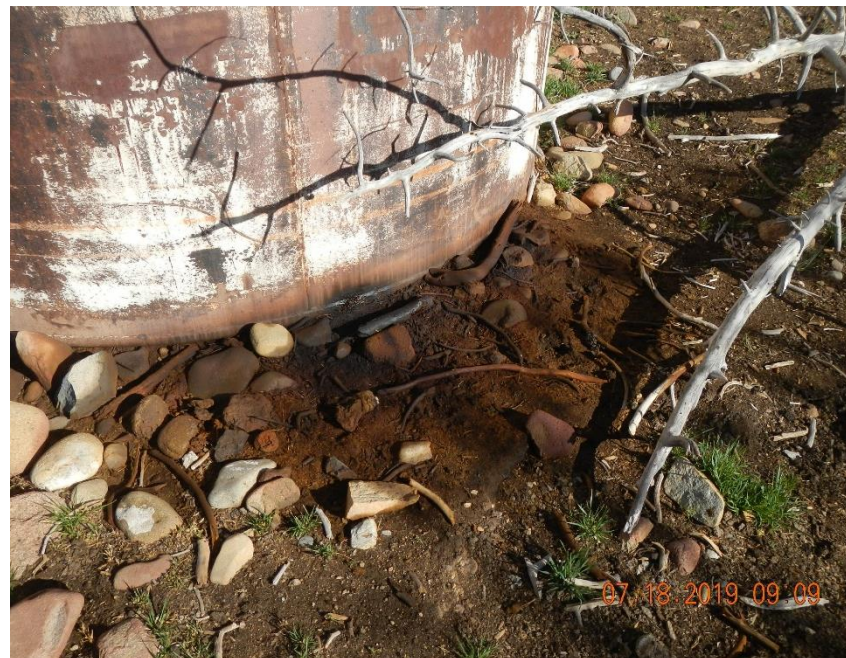
Corroded bottom seam and stained soil.
