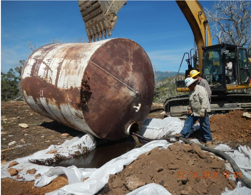
Flushing residue from AST.
