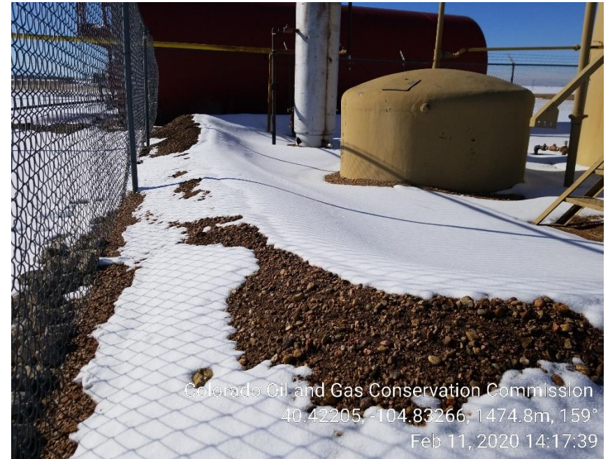
Photo 12: Inadequate berm walls
