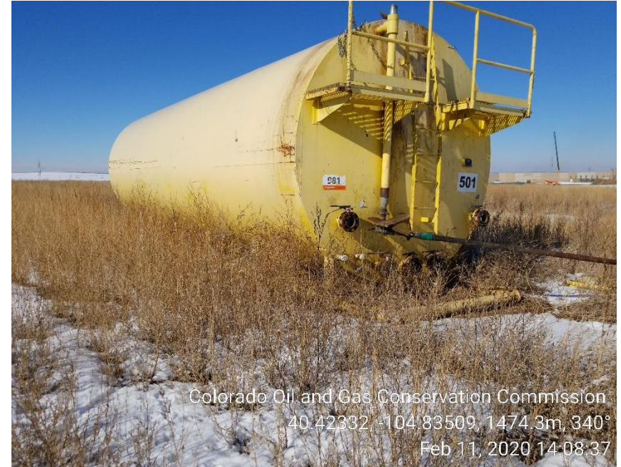
Photo 6: Maintenance tank not in containment, doesn't appear to be grounded, weeds
