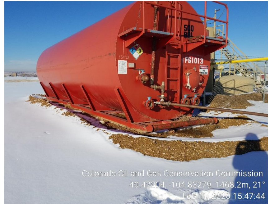
Photo 16: Tank appears to not be grounded
