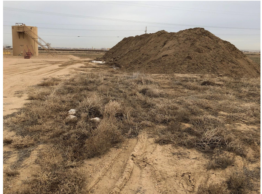
Photo 4. Photo taken from the eastern perimeter of location on January 10, 2020, facing West.. Photo depicts no ditch and berm BMPs installed throughout site; Tank battery in background. Unconsolidated soil pile on pad site may be apart of adjacent agricultural field.
