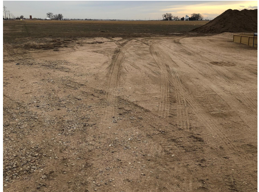
Photo 2. Photo taken from the Northwestern corner of location on January 21, 2020, facing South. Photo illustrates no ditch and berm BMP installed after interim reclamation. No current runoff issues existed at time of inspection.
