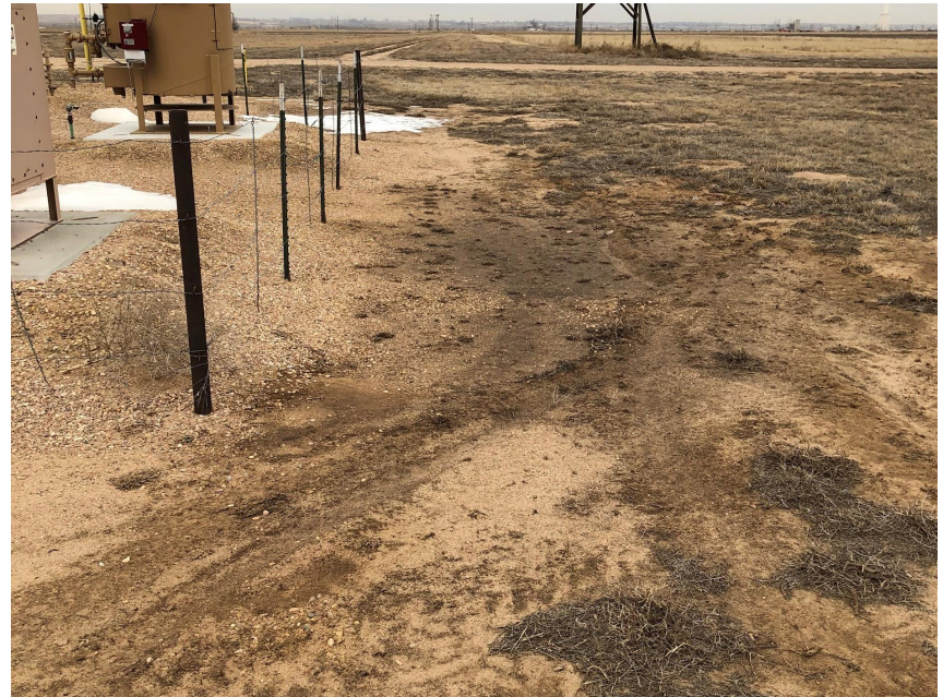
Photo 4. Photo taken from the eastern perimeter of location on January 10, 2020, facing North. Photo depicts no ditch and berm BMPs installed throughout site; interim reclamation germination will require a follow up visit.
