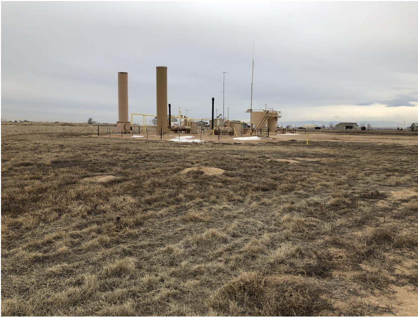
Photo 1. Photo taken from the Northern perimeter of the location on January 21, 2020, facing Southeast. Photo illustrates the completion of intermediate reclamation; however, Operator did not reinstall ditch and berm BMP at the time of this inspection. Germination in interim area was high but will require a follow up to due to high amounts of mowed weedy debris.
