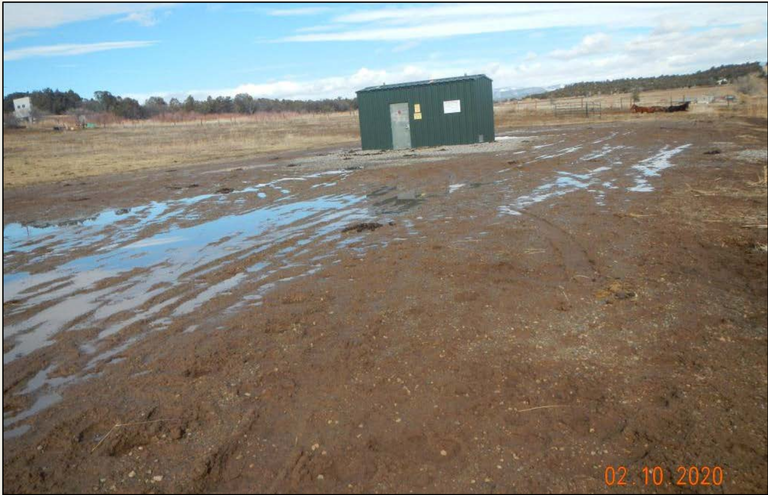
Photo 1. View of the monitoring well from the southwestern corner facing center.
