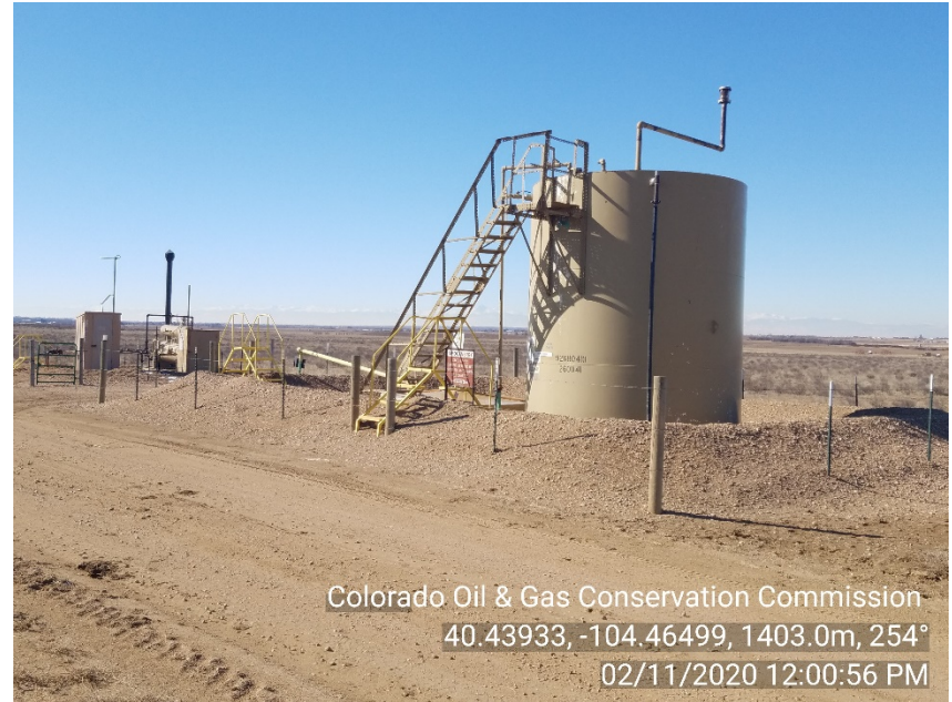
Photo #2 State 23-32 Battery site Inactive | Shut-down Formerly served State 14-32, 24-32 ( Plugged & Abandoned | PA )
