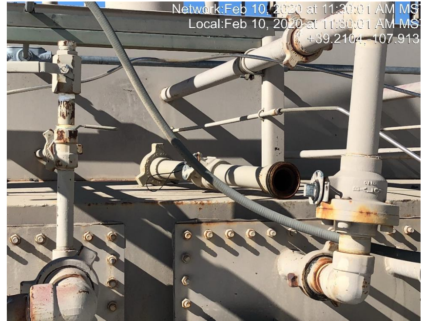
Photo #0548 Unused equipment on top of separator.
