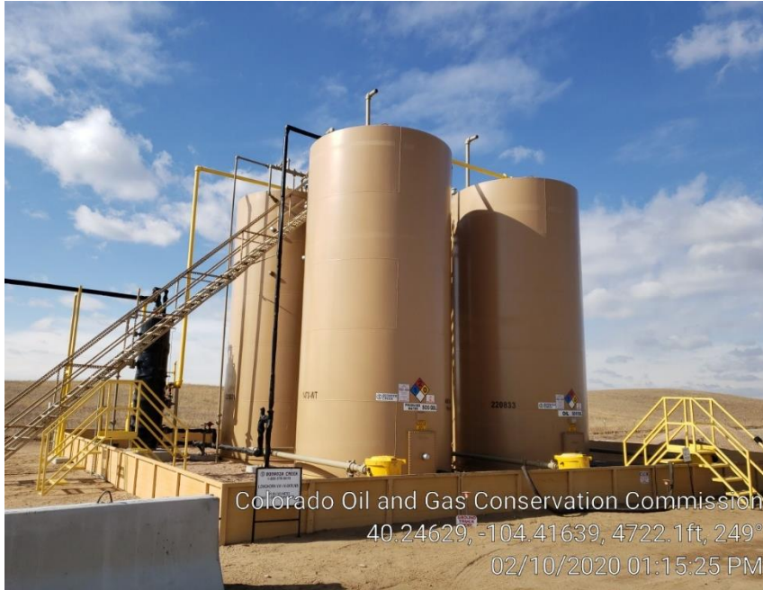
Photo #2 Tank Battery
