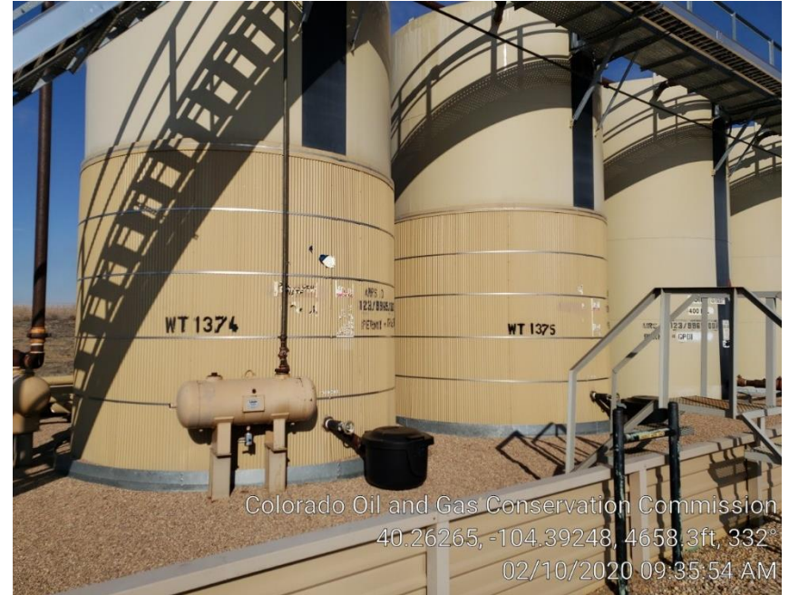
Photo #7 Capacity & Placards "NFPA" not legible on water tanks.
