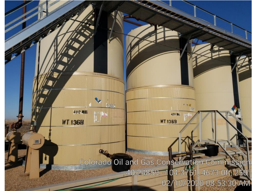
Photo #8 Placards "NFPA" not legible on water tanks.
