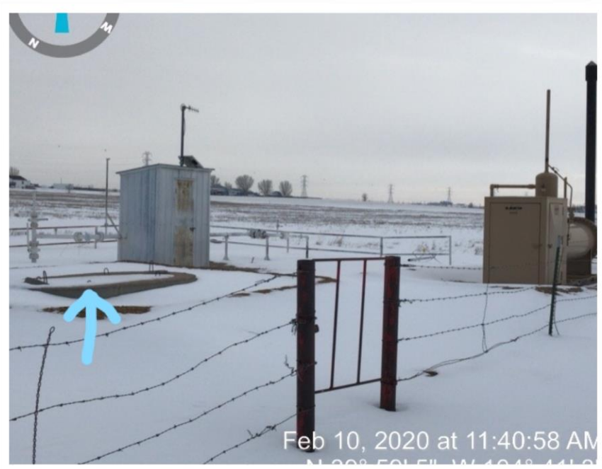
Photo #2 Unmarked produced water tank, separator & meter run
