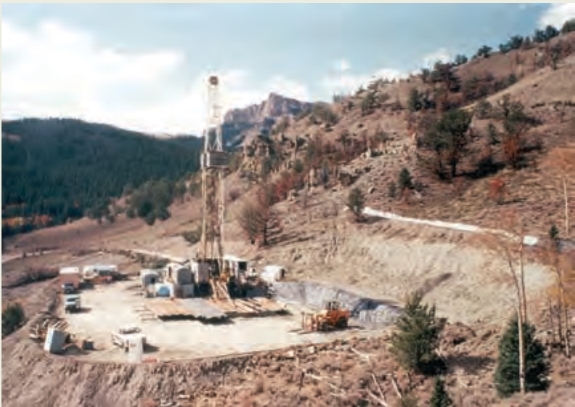
The well pad and access road are constructed to the minimum size necessary to safely conduct drilling and completion operations.
