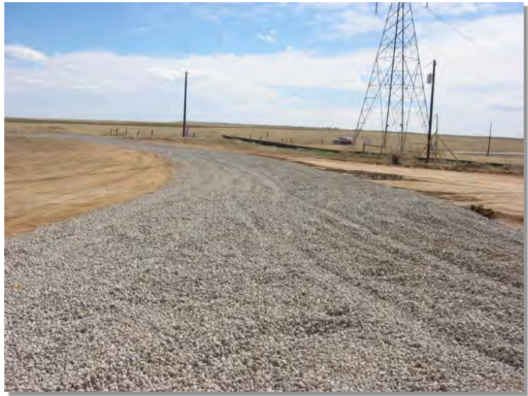
Photograph SCR-1. Stabilized construction roadway.
