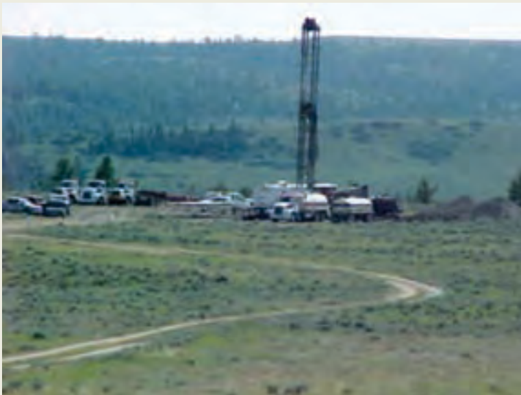
A minimum disturbance, primitive, two-track road winds its way to a drilling operation. To further reduce disturbance, most of the well location has not been stripped of vegetation or topsoil.
