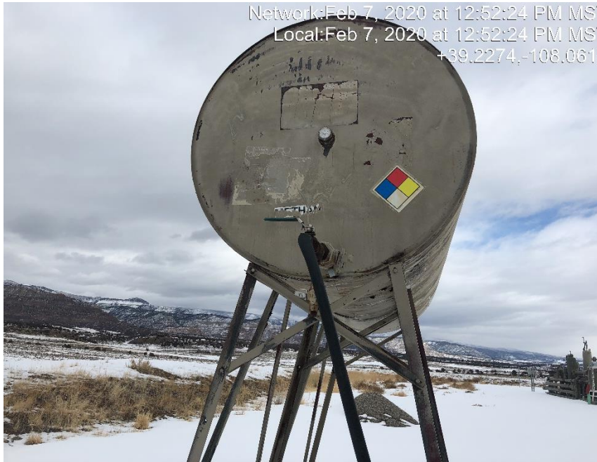
Photo #0545 1000 gallon tank contents and NFPA labels weathered and not legible.
