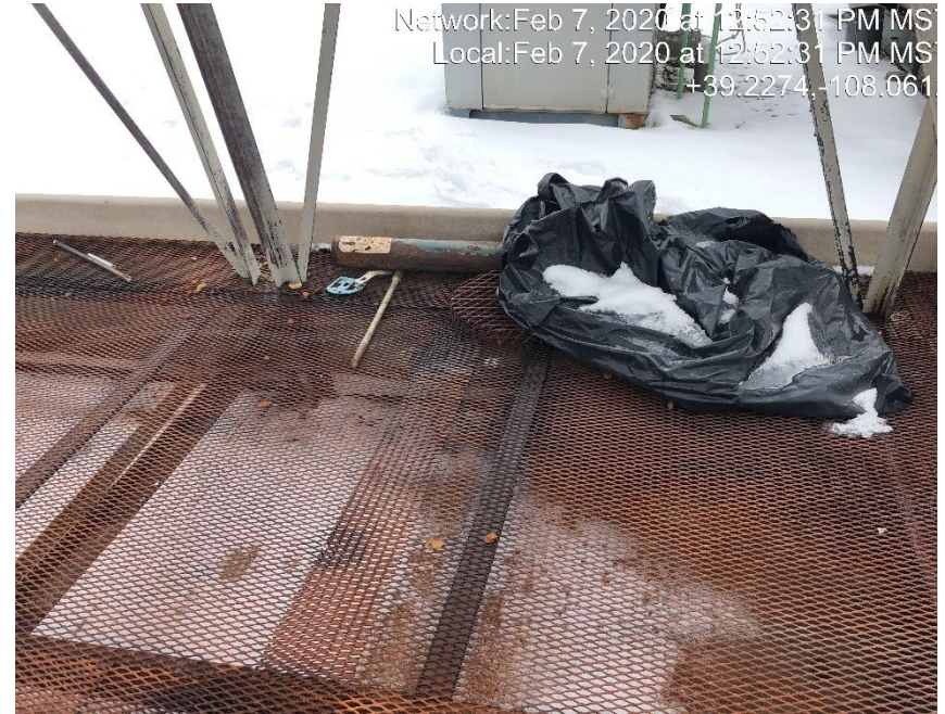
Photo #0546 Unused equipment and debris in 1000 gallon tank containment.
