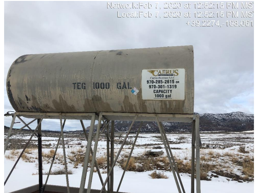
Photo #0544 1000 gallon tank contents and NFPA labels weathered and not legible.
