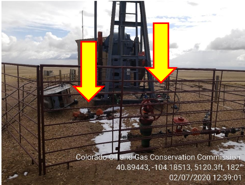
Photo 3 – Unused Wellhead parts
