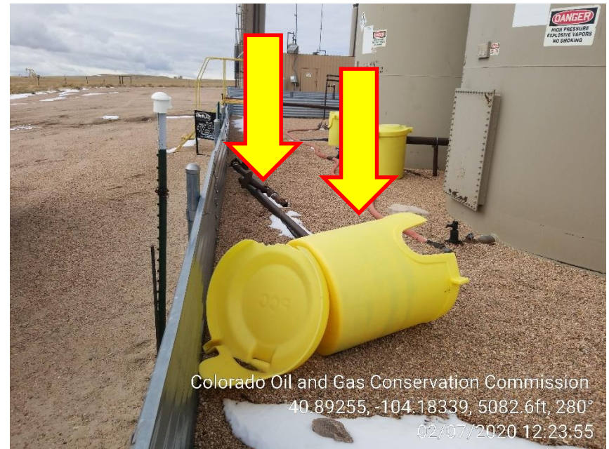
Photo 4 – Unused Loadline Bucket and 3" pipe
