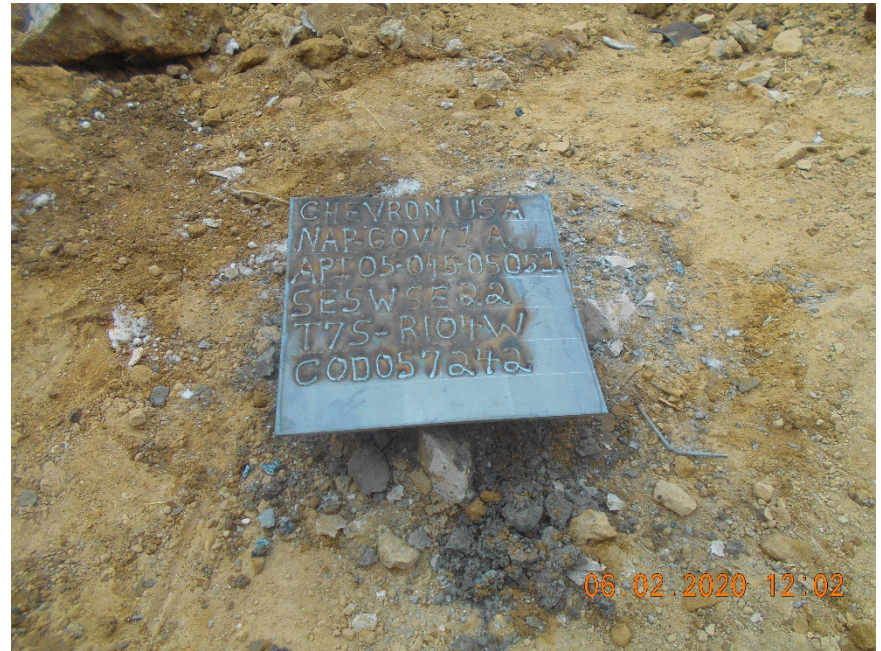
Information plate welded on cut casing prior to burial.
