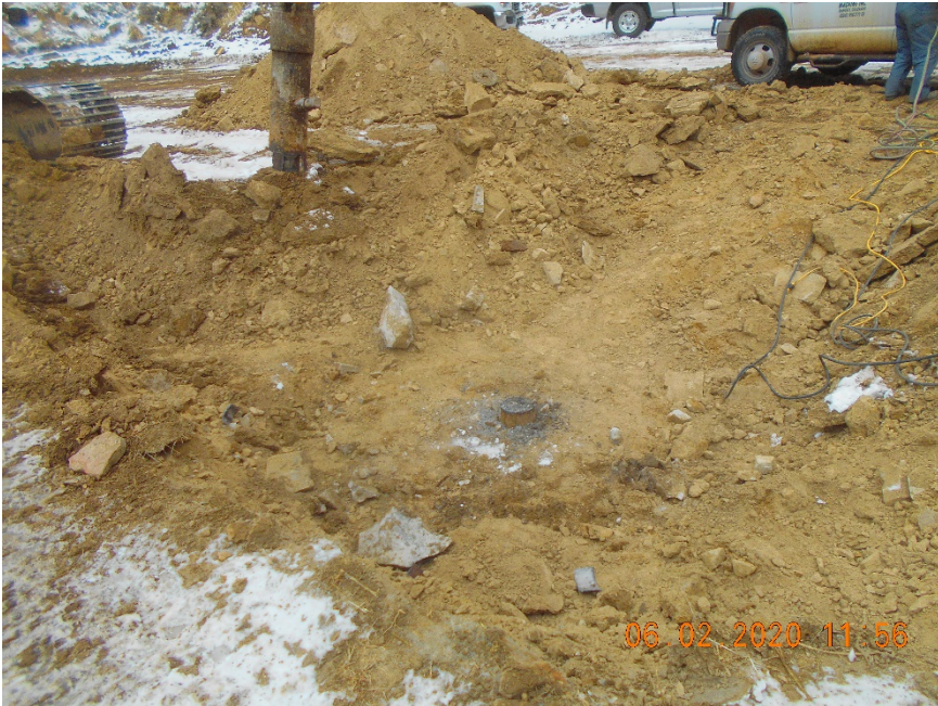
Removal of wellhead after final plugging operations
