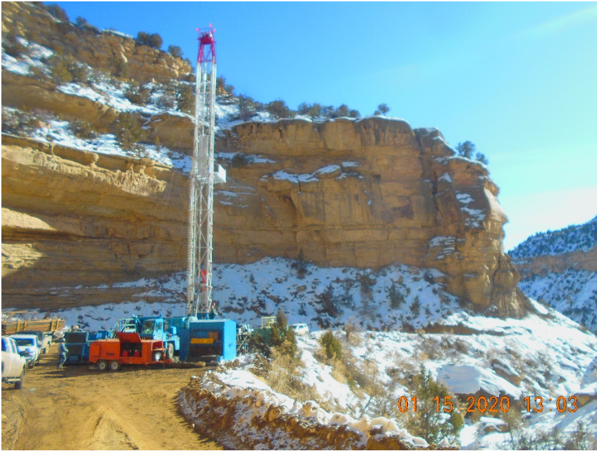
Rig on Location.
