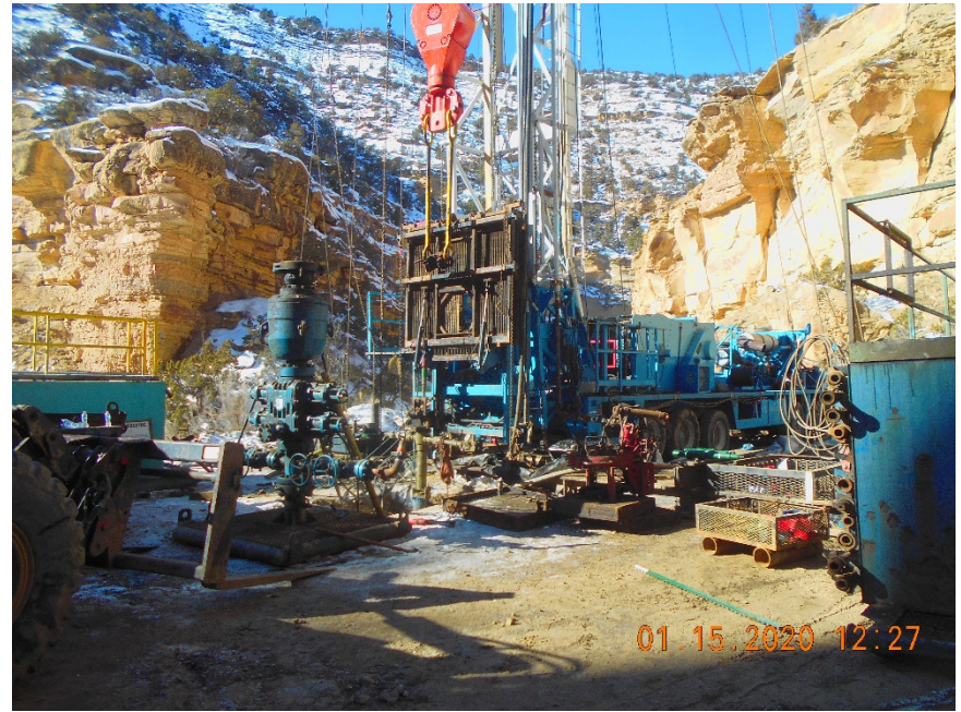
Rig up on wellhead to begin plugging operations.
