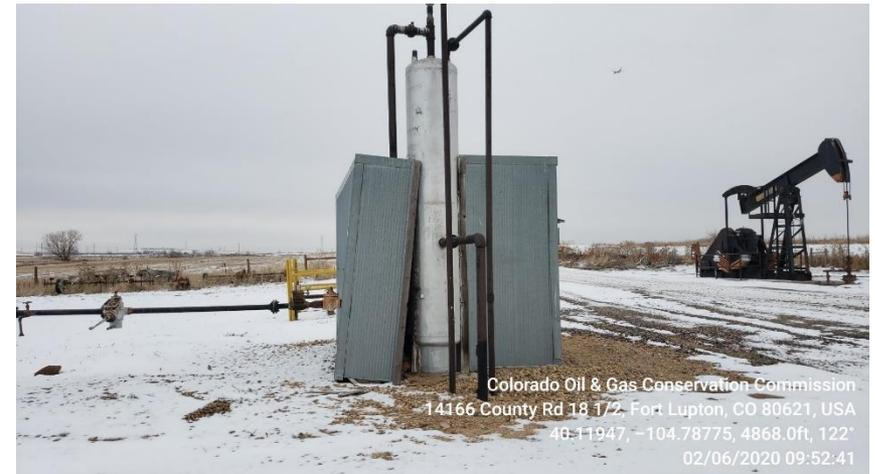
**Photo 9 Horizontal heated separator**
