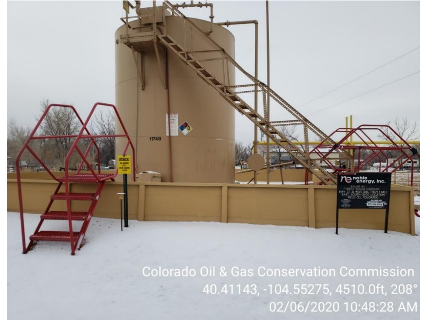
Photo 2 Tank Battery
