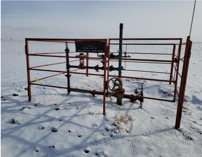
Photo #1 Well & Sign
