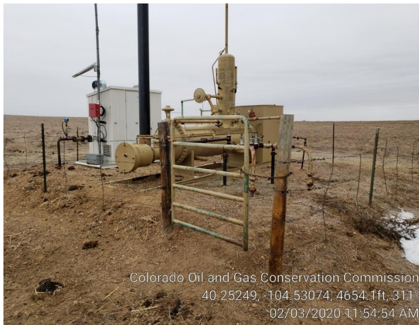
Photo #3 Separator, Meter Run & No Weeds
