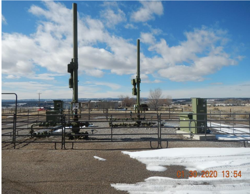
Linear rod pumps on both well heads.
