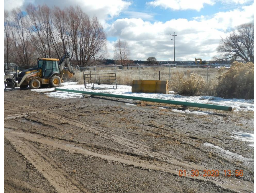
Joint of 6" steel pipe on location. Equipment in background is backfilling excavation for Spill/Release Point ID #470891.
