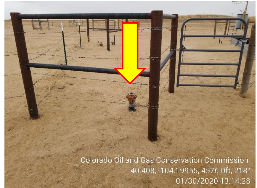
Photo 4 – Unmarked Risers
