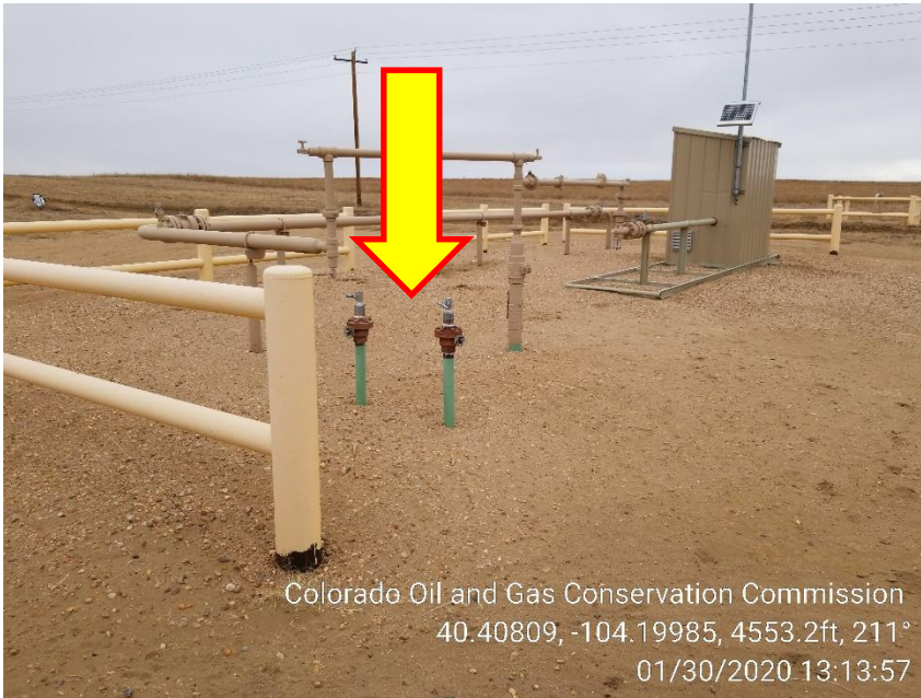
Photo 3 – Unmarked Risers
