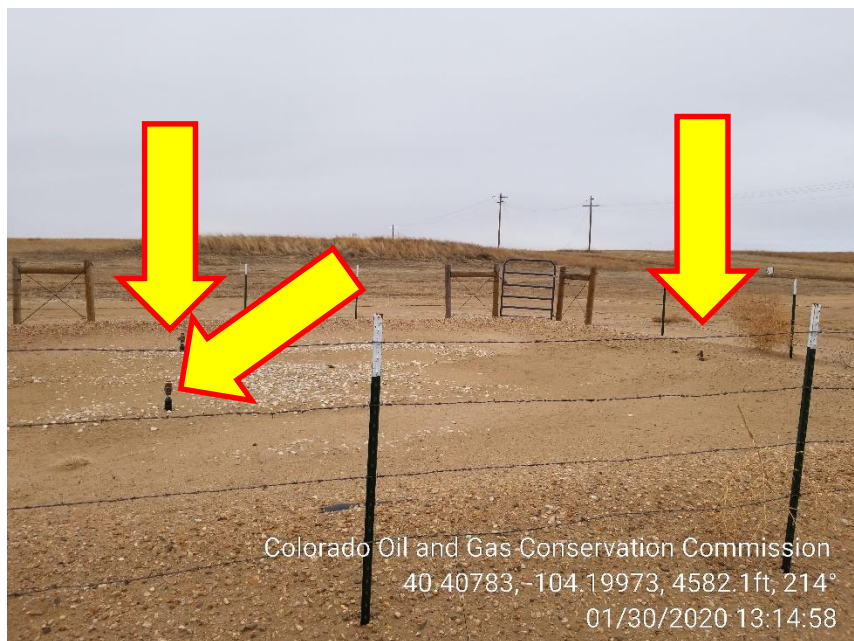
Photo 5 – Unmarked Risers
