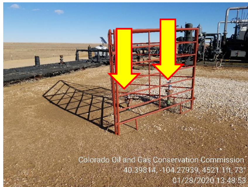
Photo 4 – Unmarked Risers; west of Compressors
