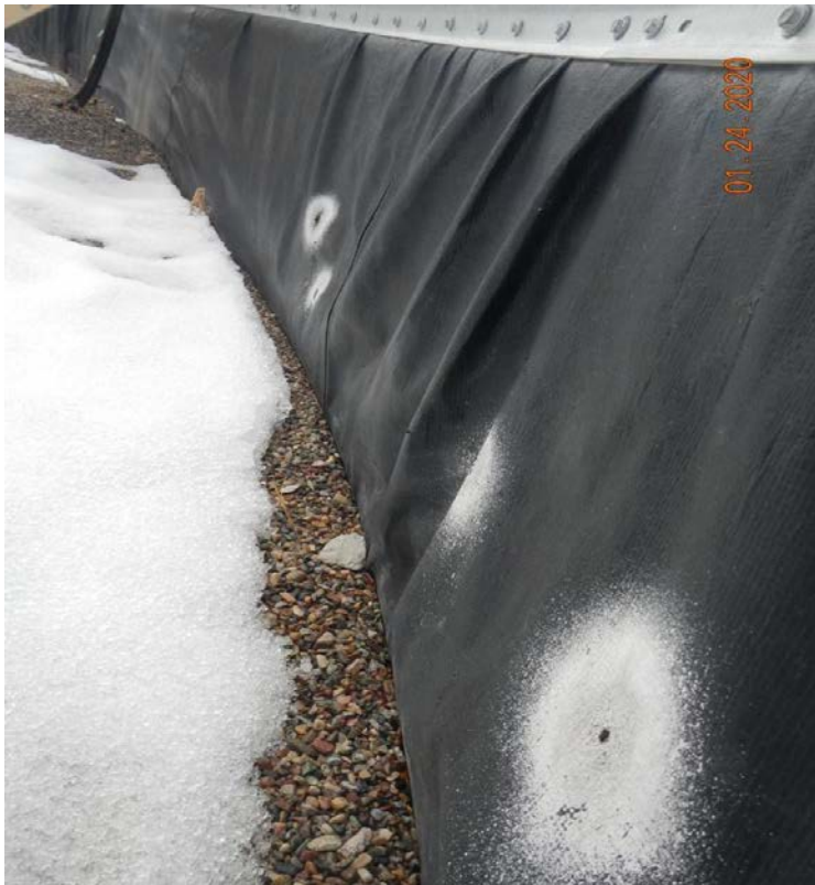
Photo#4: What appeared to be failed repairs of pinholes observed in battery liner.
