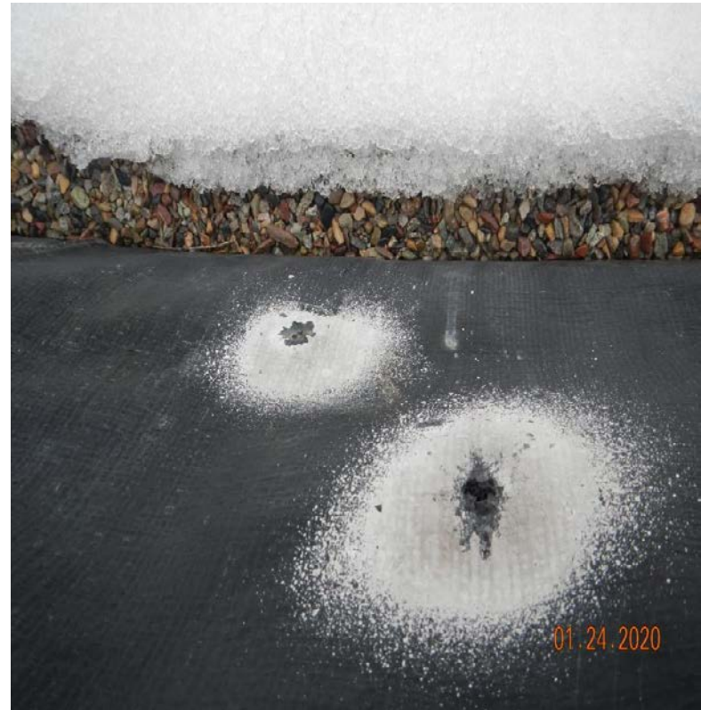
Photo#5: What appeared to be failed repairs of pinholes observed in battery liner.
