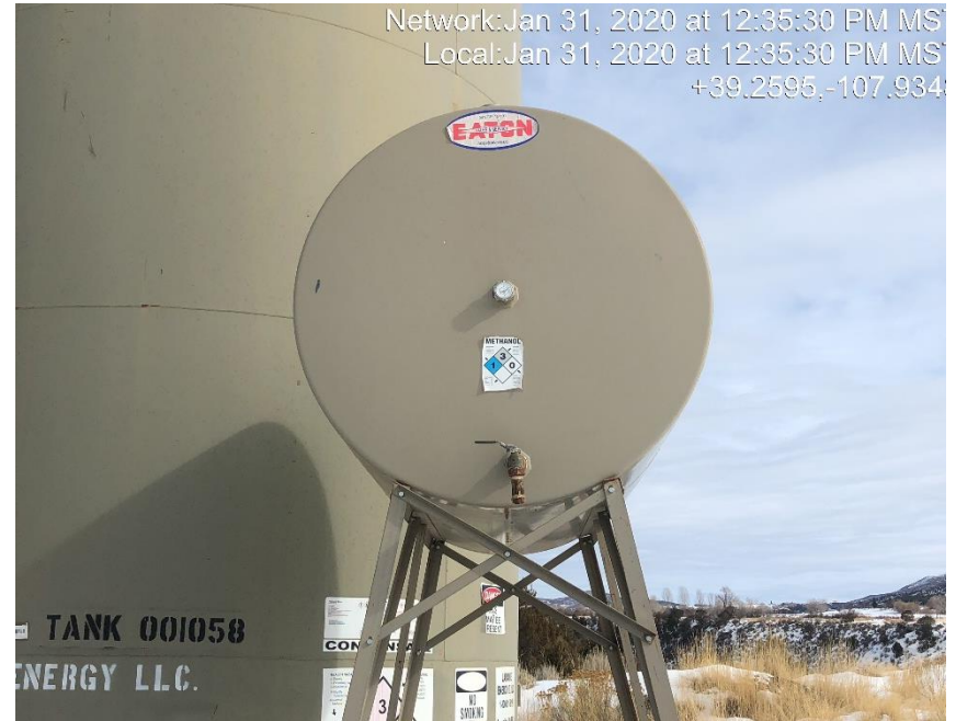
Photo #0514 Tank capacity not labeled on methanol tank.
