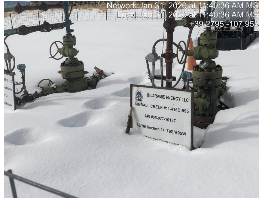
Photo #0510 Unused bumper spring, bull plugs and gauge at wellheads.
