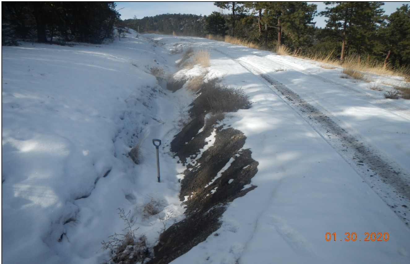
Photo 1. Facing southwest along the access road. The side of the road has eroded. This area needs to be repaired and BMP's need to be installed.
