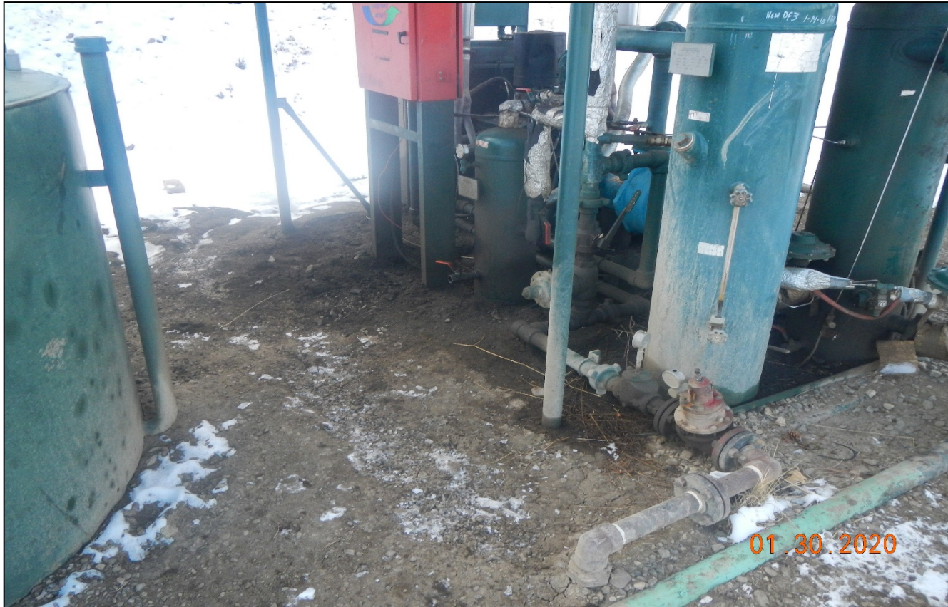
Photo 3. There is oil stained soils near the tank and separator. This needs to be cleaned up.
