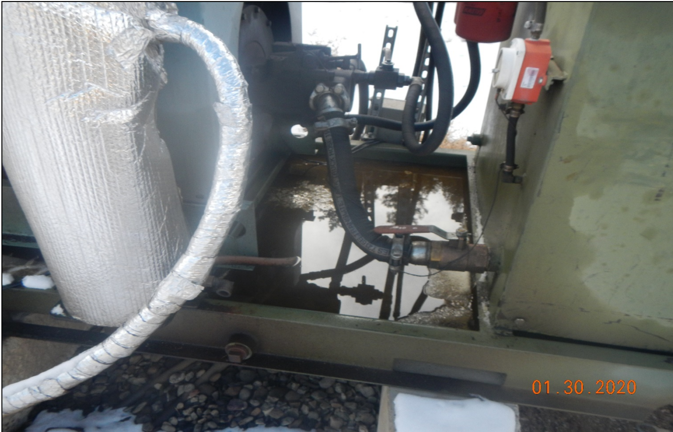
Photo 4. There is oily water In the engine skid.
