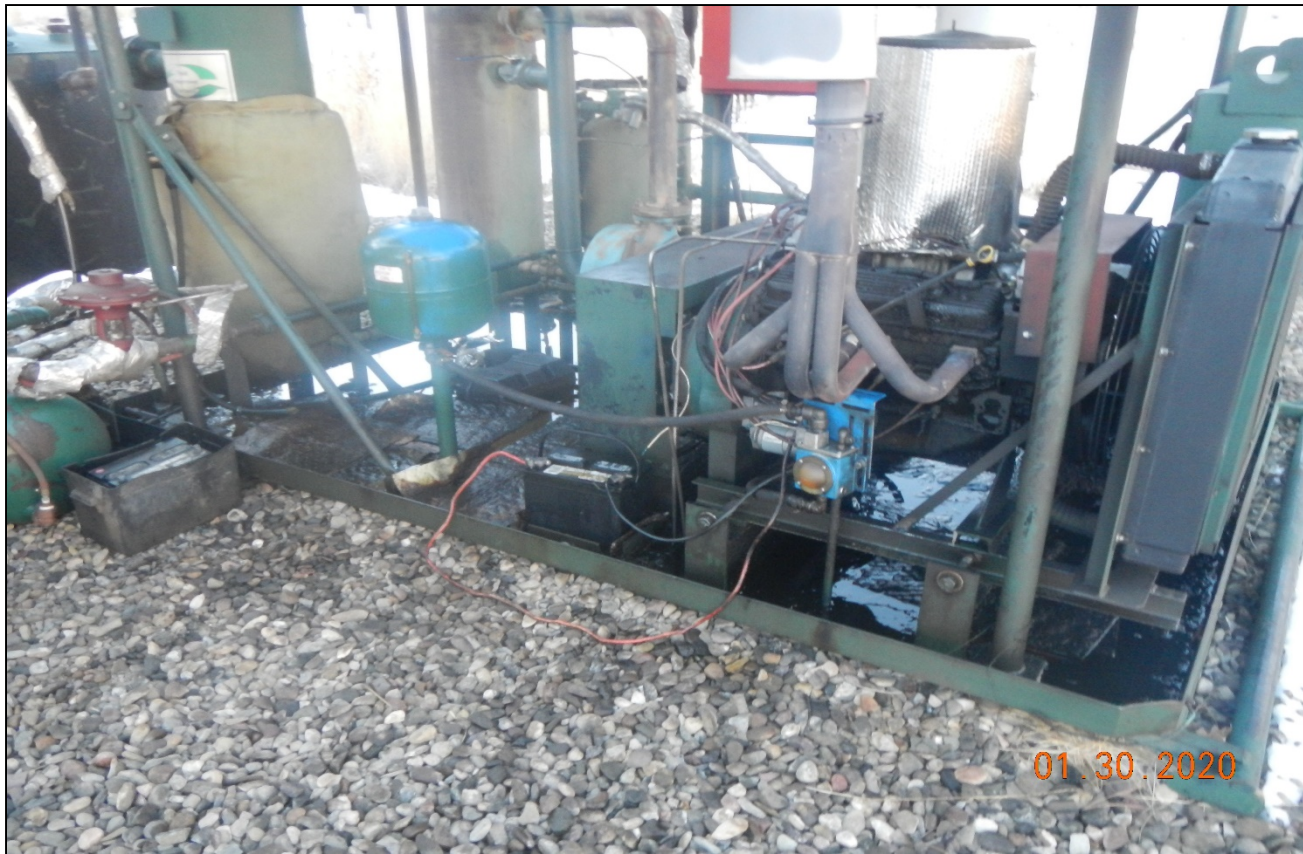
Photo 2. There is oily waste in the engine skid that needs to be cleaned up.
