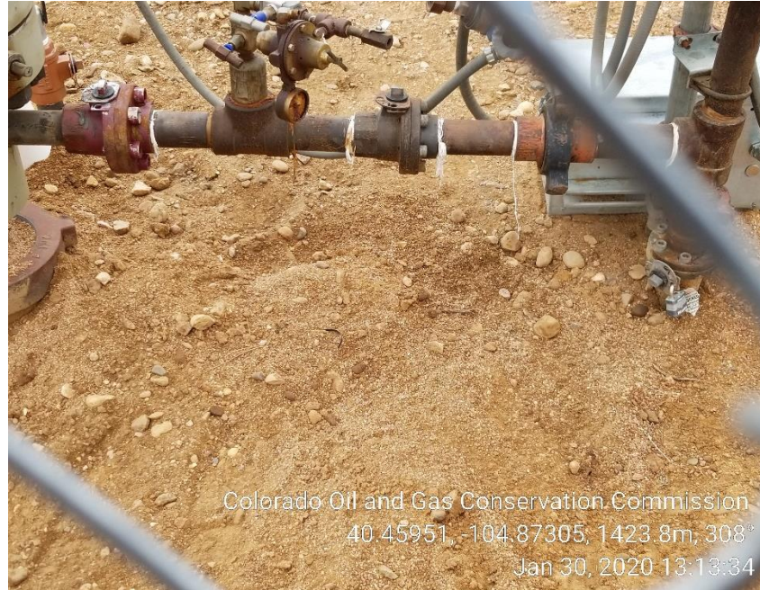
Photo 3: Stained soil removed
