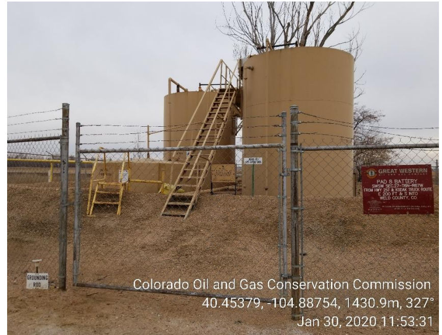
Photo 2: Tank Battery
