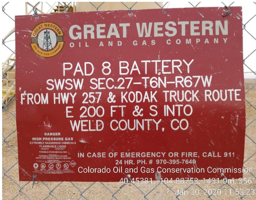
Photo 1: Tank Battery Sign
