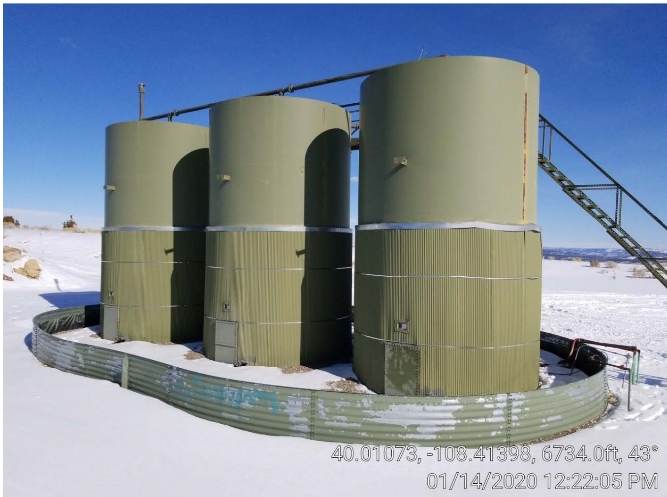
Photo 4. Tank battery.
