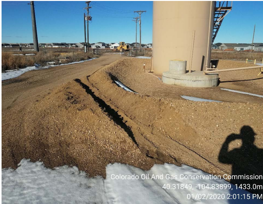
Crude oil tank berm on 1/2/2020
