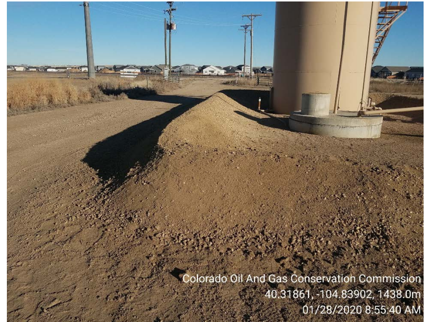
Crude oil tank berm on 1/28/2020
