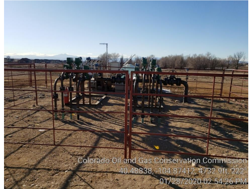
Photo #7 Gas Lift for South Production Wells
