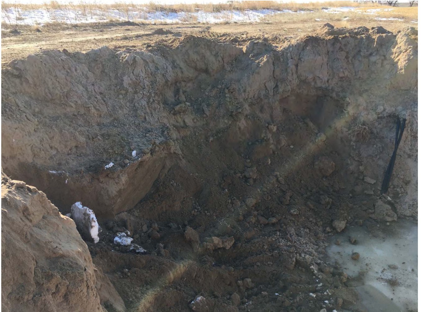
South wall following excavation to remove additional oily soils 12/10/19
