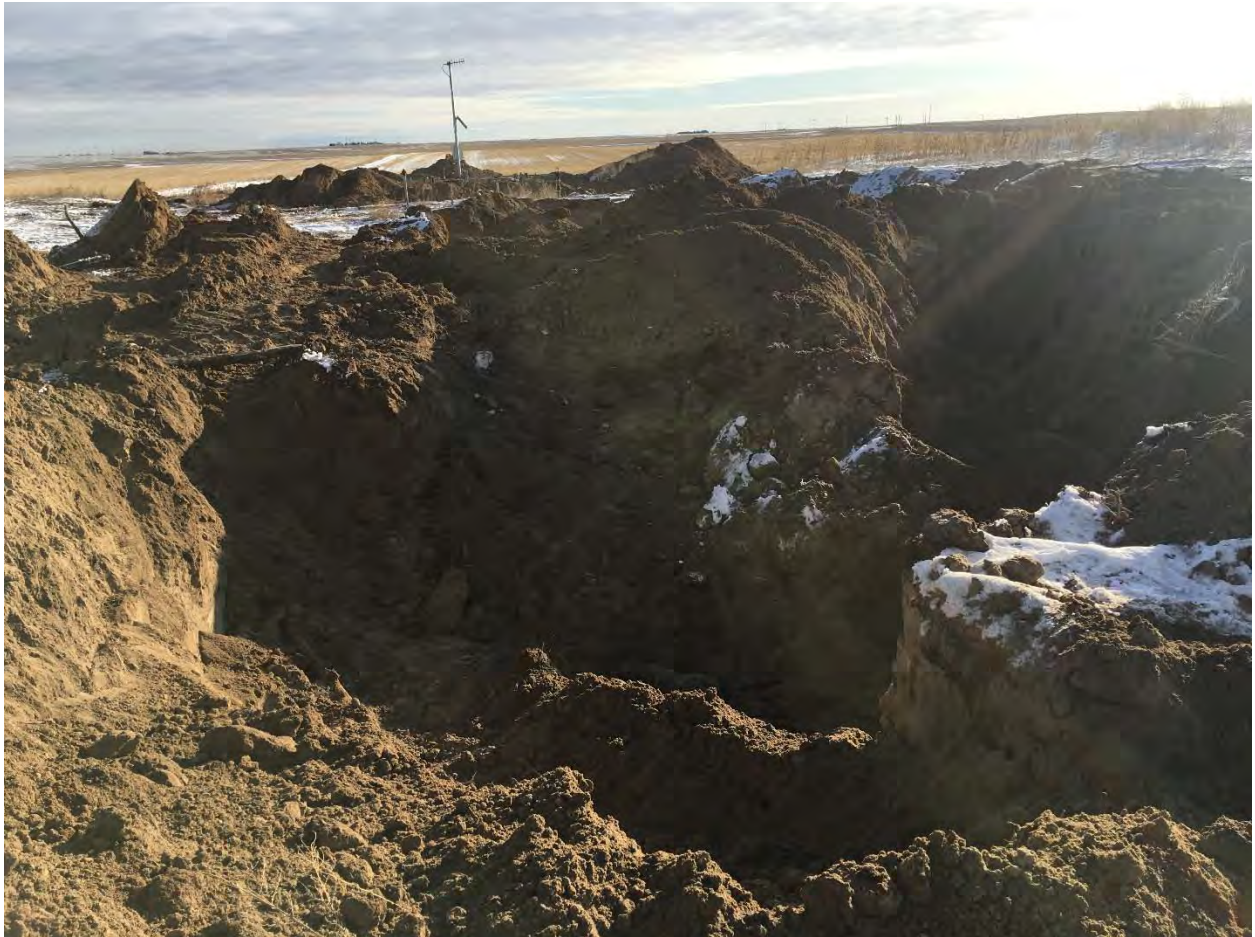
Heater treater excavation where failed sample HT was excavated and replacement sample HT @ 4' was collected, Looking East 12/17/19
