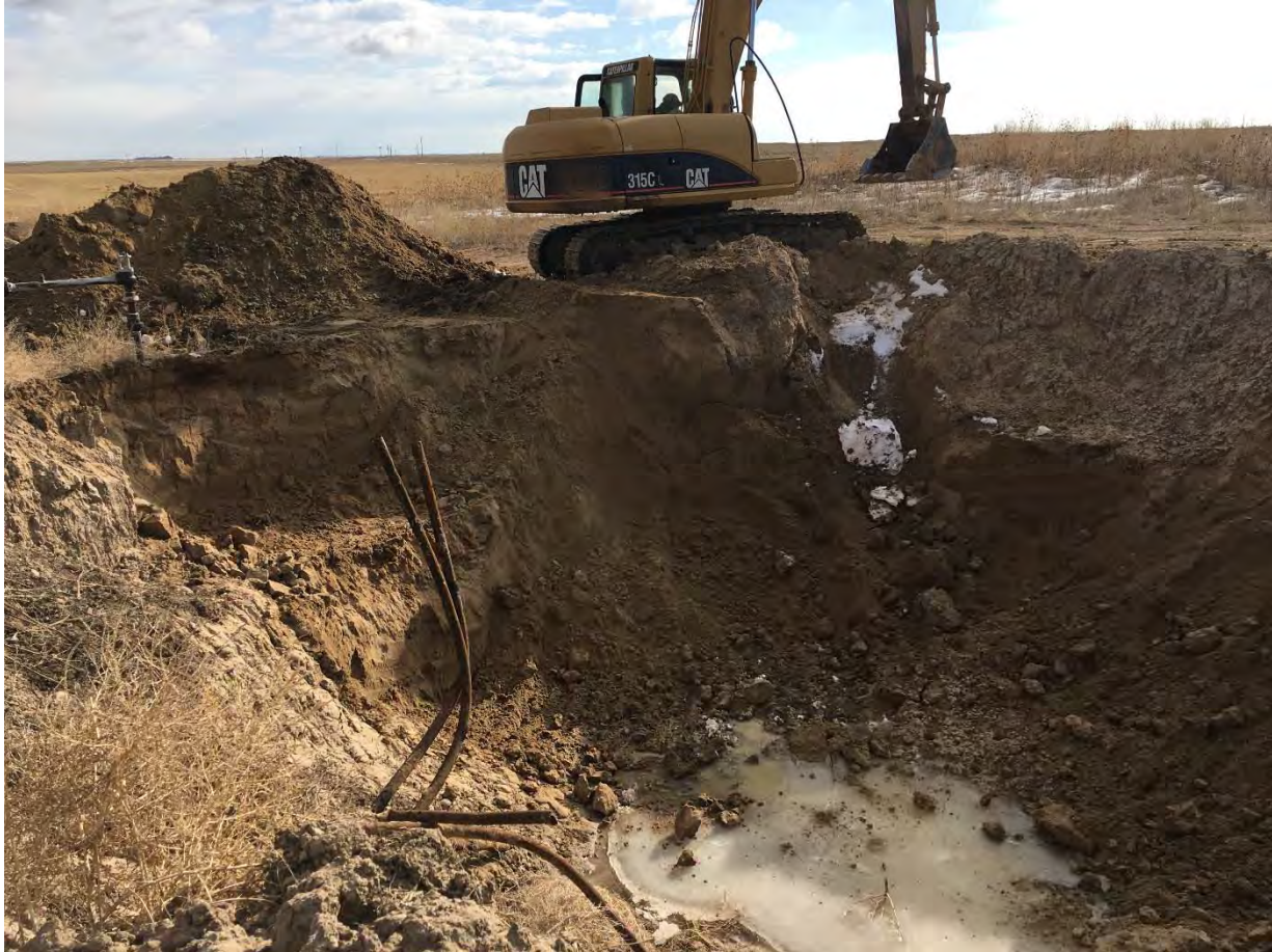
Excavation to remove additional oily soils 12/10/19
