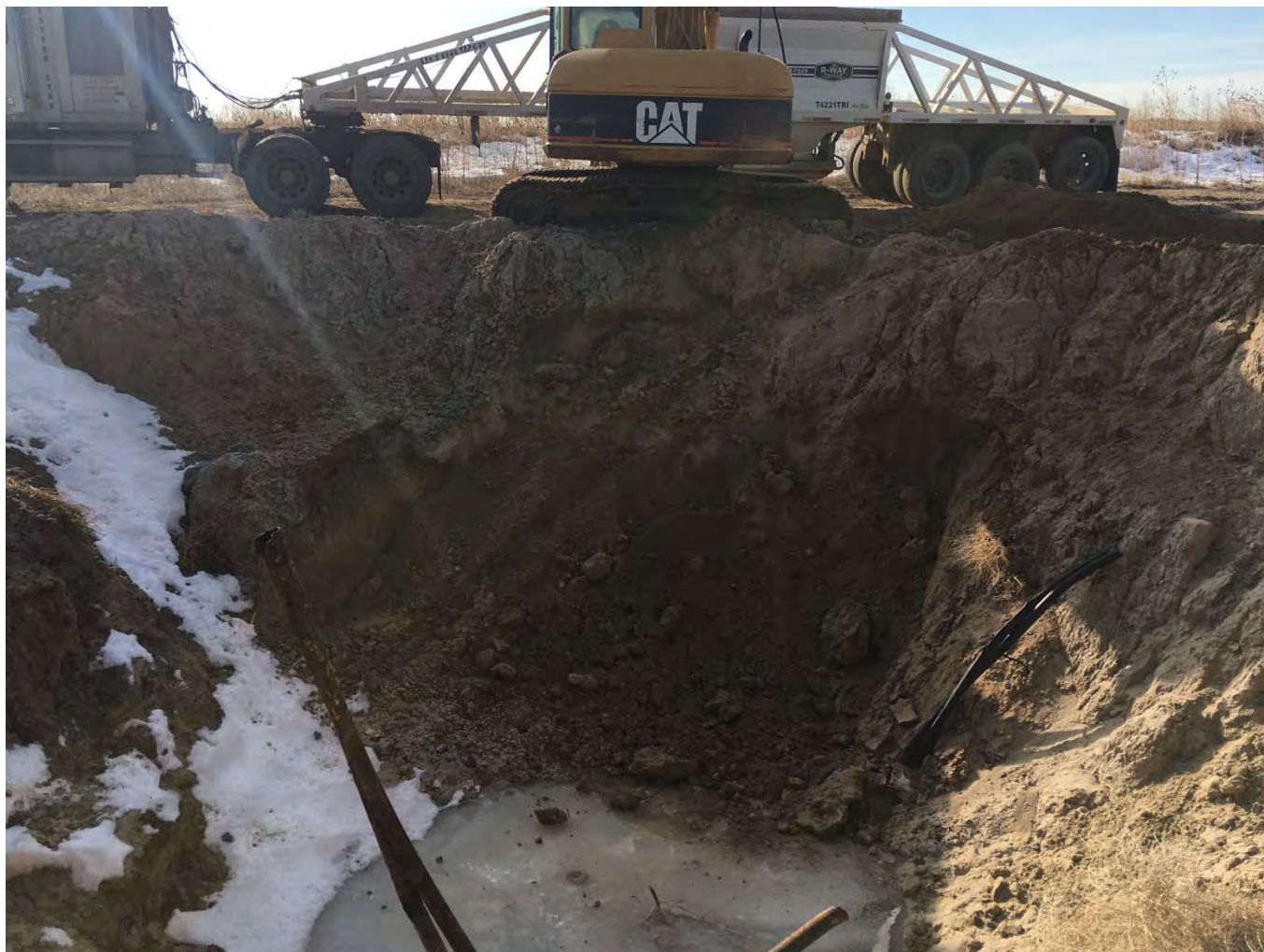
Impacted soils being loaded for disposal 12/10/19
