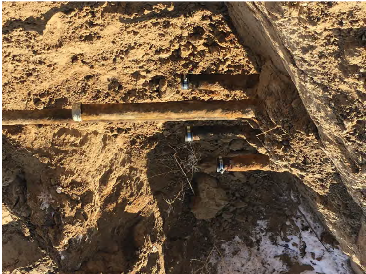
Capped piping in the PTA area 12/17/2019
