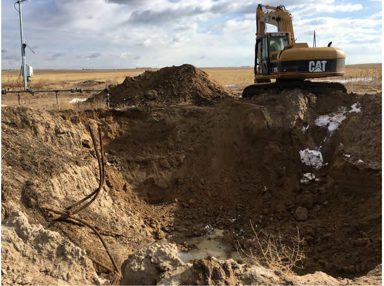
Excavation to remove additional oily soils 12/10/19
