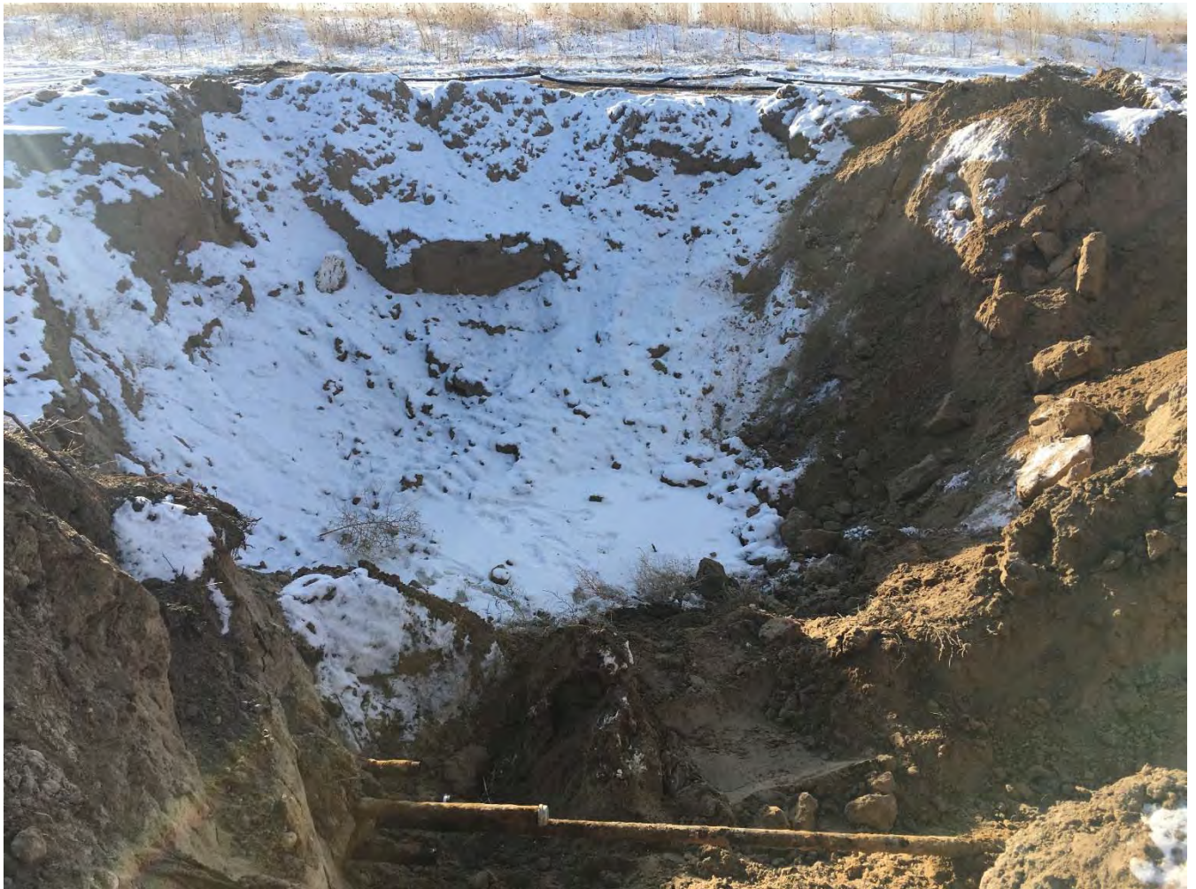
South wall of Pit excavation where piping has been uncovered and capped looking South 12/17/19
