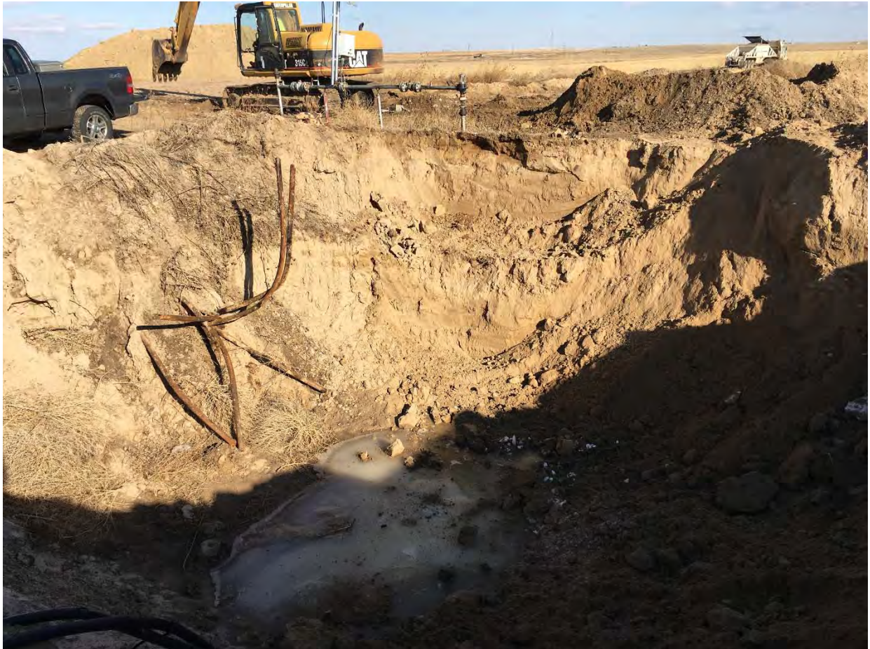
East wall following excavation to remove additional oily soils 12/10/19
