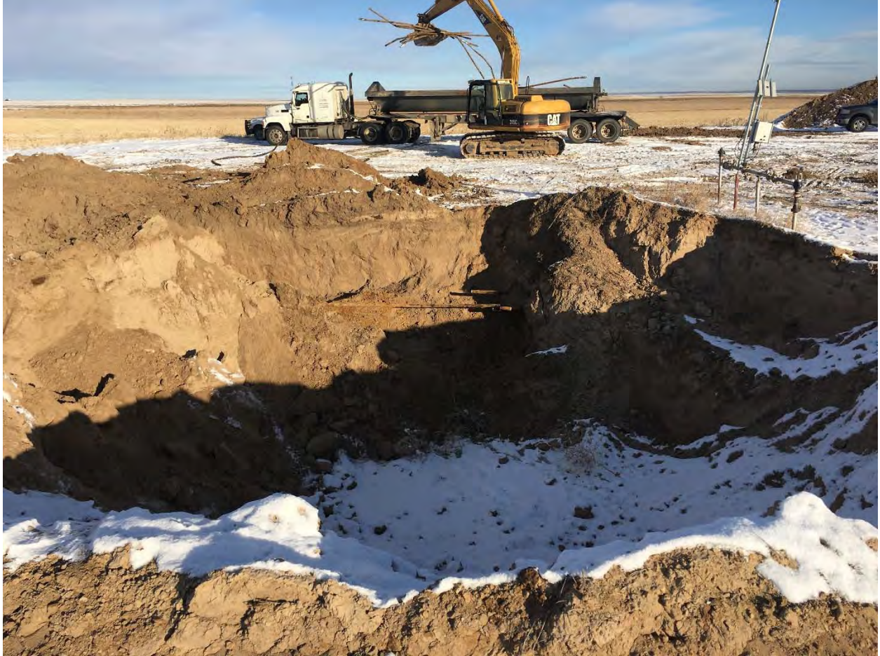
North wall of Pit excavation where piping has been uncovered and capped Looking North where piping is being loaded for disposal 12/17/19
