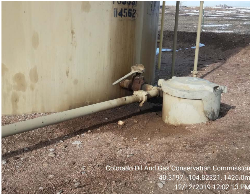
Load valves and stained soil on 12/12/2019
