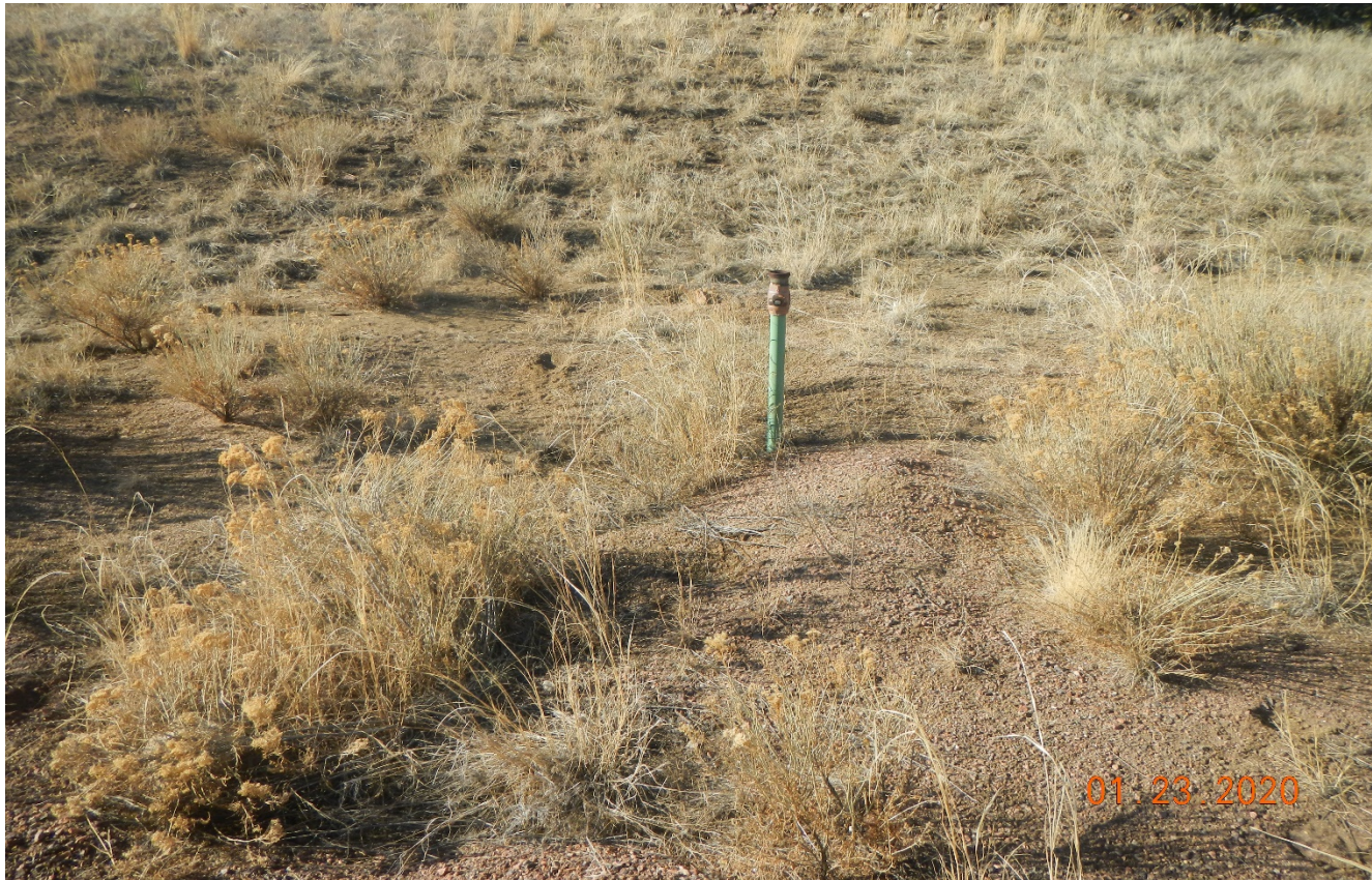
Photo 5. The pipe riser at the west side of the location has no LO/TO.
