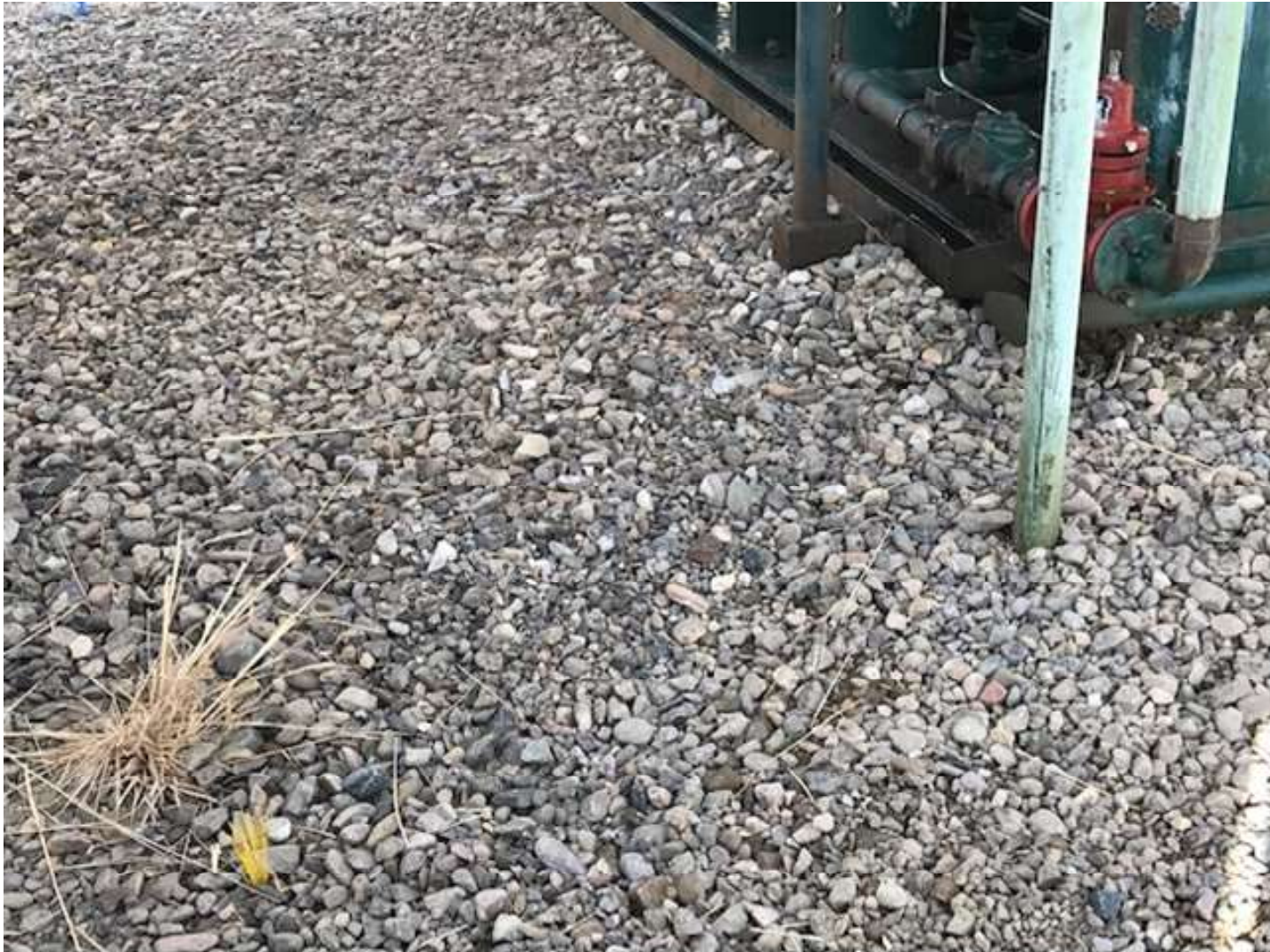
PHOTO 5: THE IMPACTED SOIL NEXT TO THE LIQUID RING COMPRESSOR WAS REMOVED FROM THE LOCATION.
