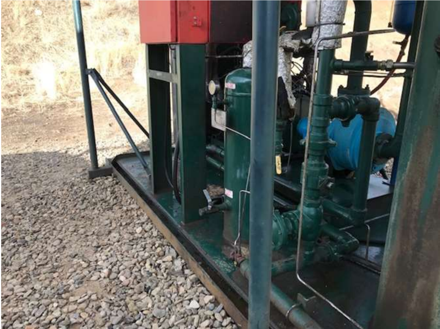
PHOTO 2: THE SKID OF THE LIQUID RING COMPRESSOR WAS CLEANED AND THE FLUID ACCUMULATION WAS REMOVED FROM THE RESERVOIR.
