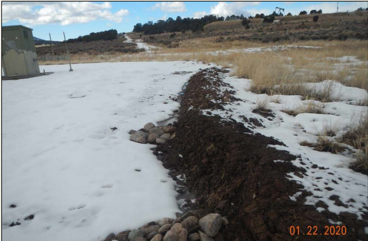
Photo 2. View of berm installed within the northern project area. Berm is not stabilized.
