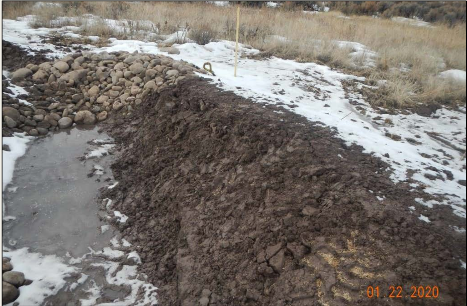
Photo 5. View of silt trap installed within the western project area. Geotextile fabric not in place. Insufficient rock armoring.
