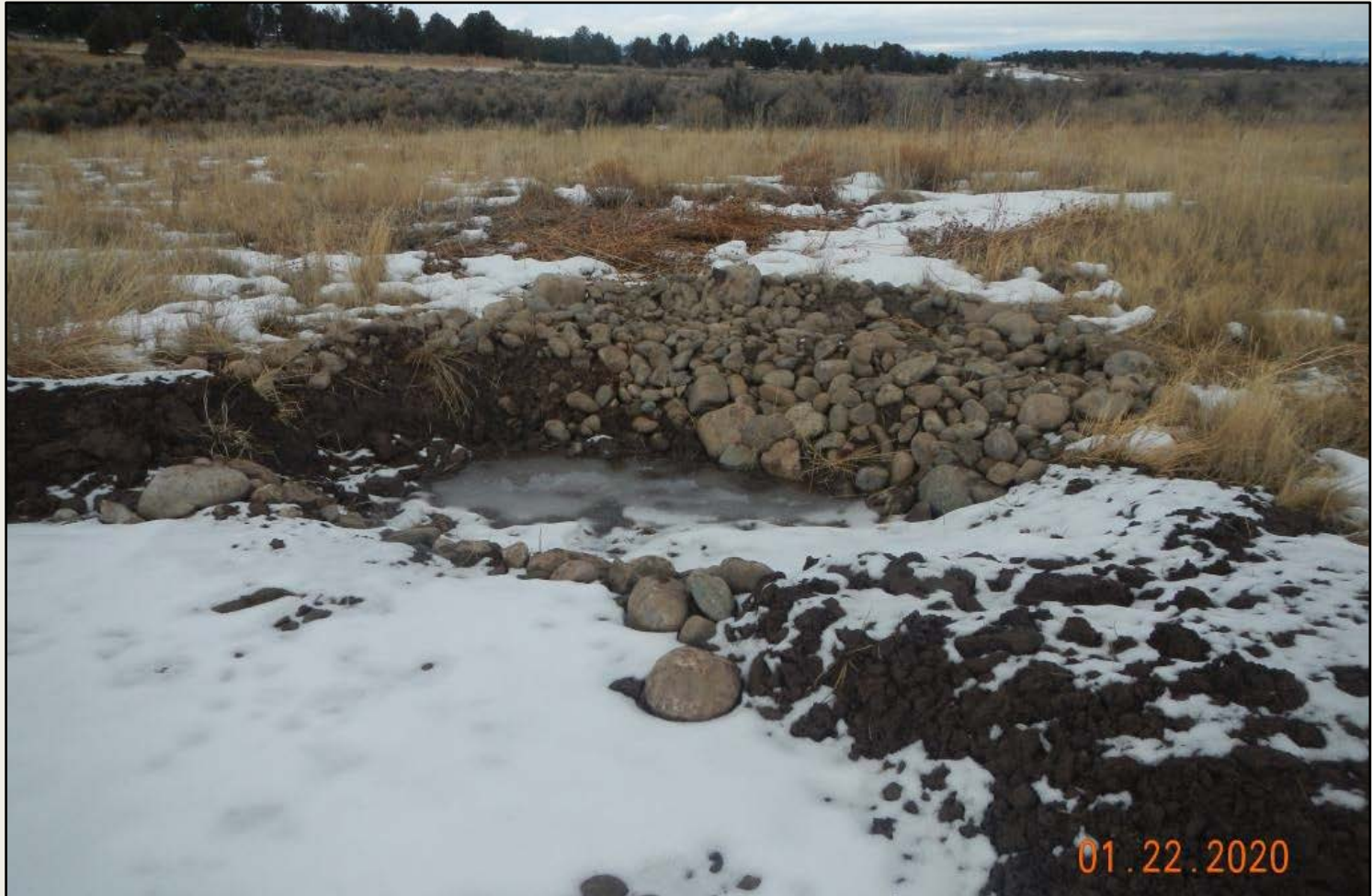
Photo 1. View of stormwater controls installed within the northern project area. Cobble rock at outlet is not adequate outlet structure. Bare soils are not stabilized.
