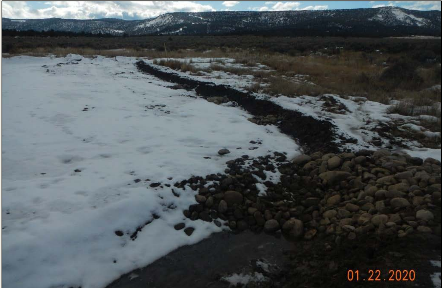
Photo 4. View of berm installed within the southwestern project area. Bare soils not stabilized, seed bed not prepared and seed not incorporated.
