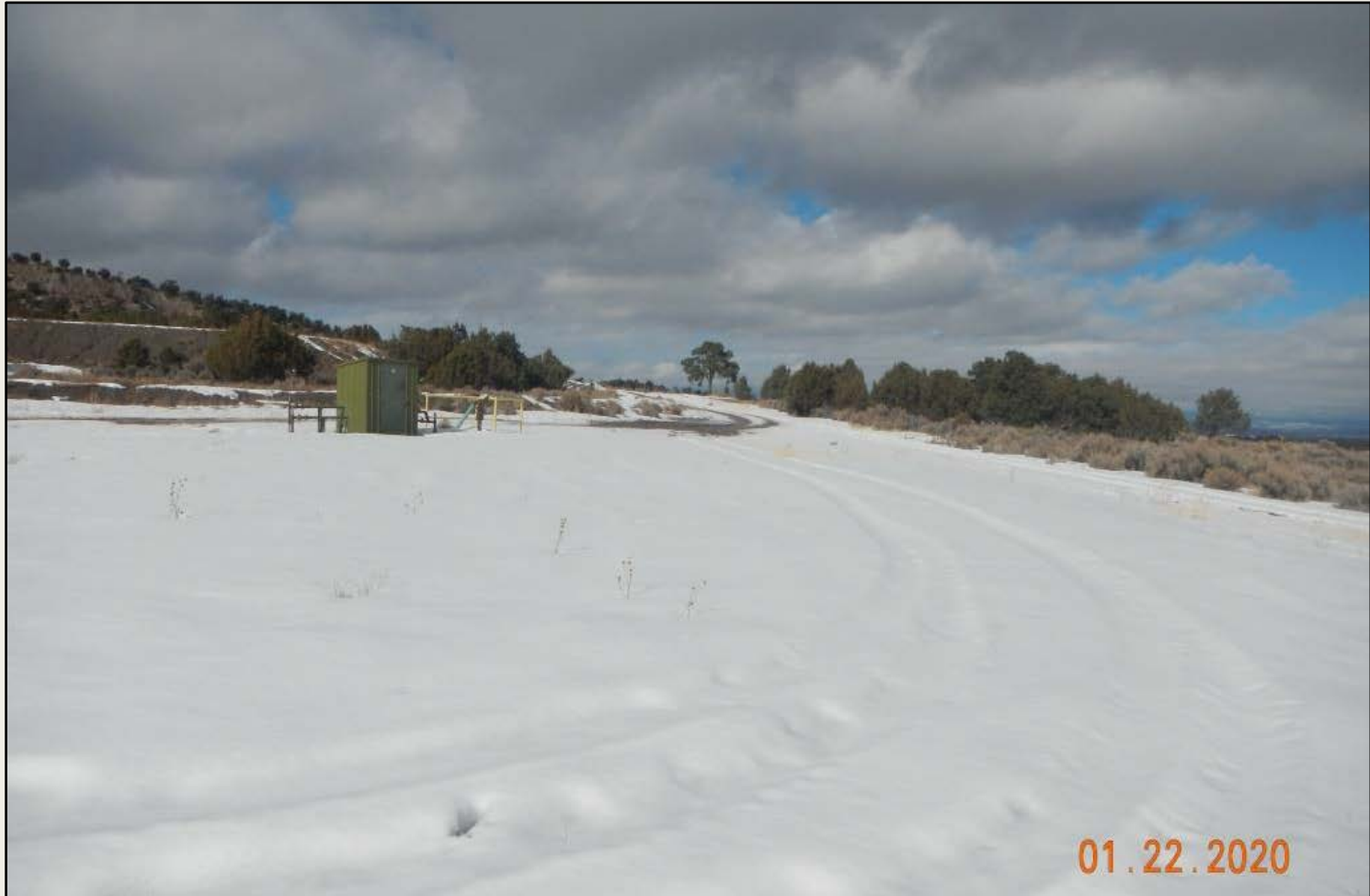
Photo 2. View of the eastern project area from the southeastern portion facing northward. Although snow covered, it is apparent that revegetation is not conducted and erosion/stormwater controls are not installed.
