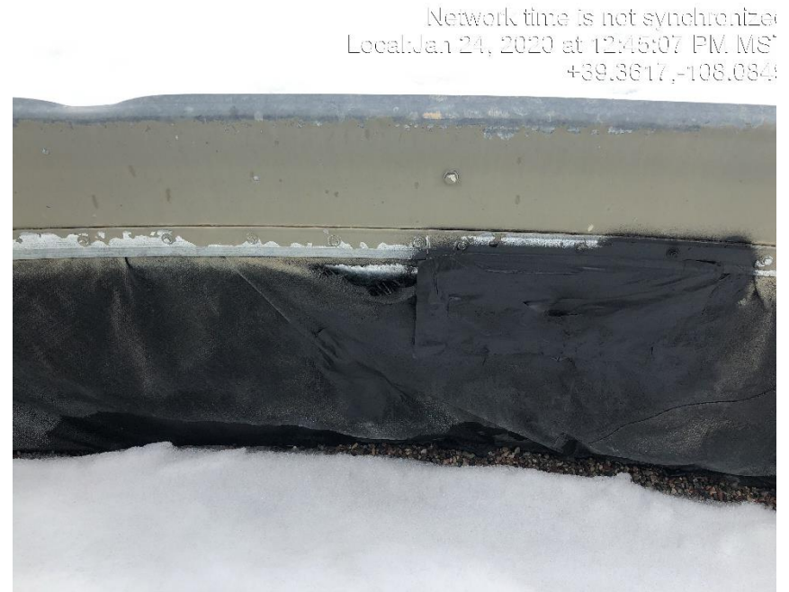
Photo #0466 Multiple holes in tank containment liner.
