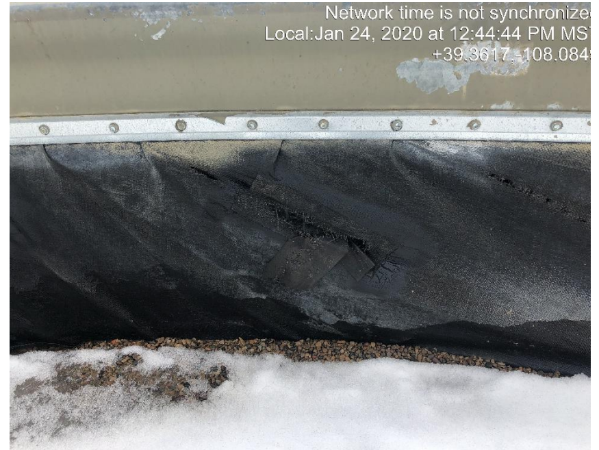
Photo #0464 Multiple holes in tank containment liner.
