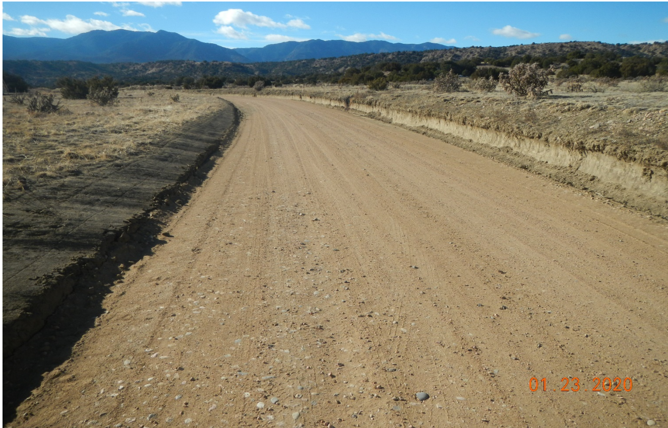
Photo 2. Facing west further along the road. Road has been repaired.
