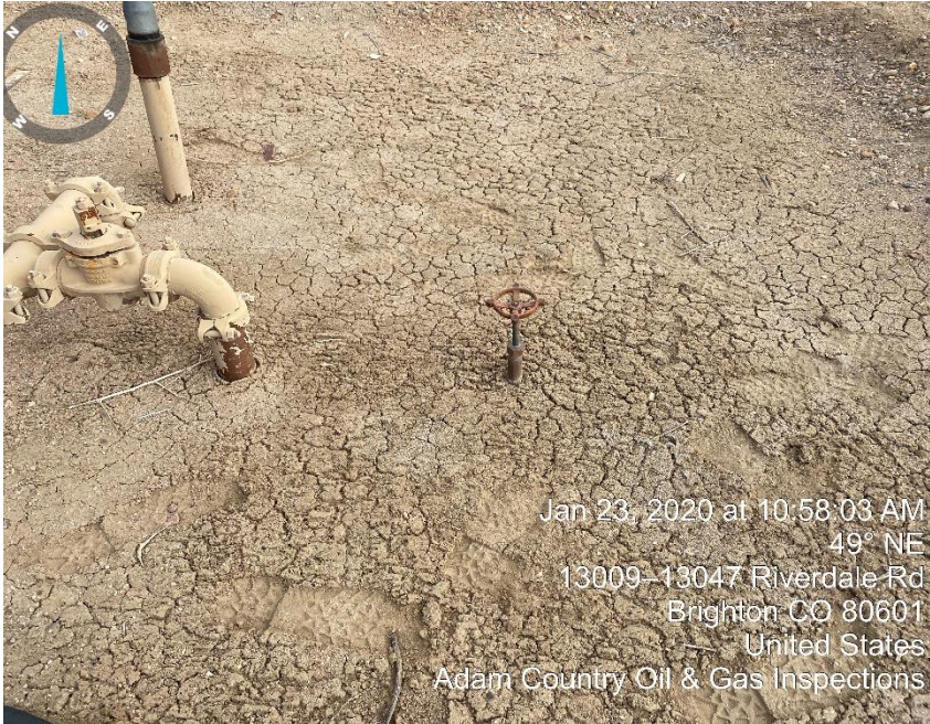
Photo #11 Unmarked riser
