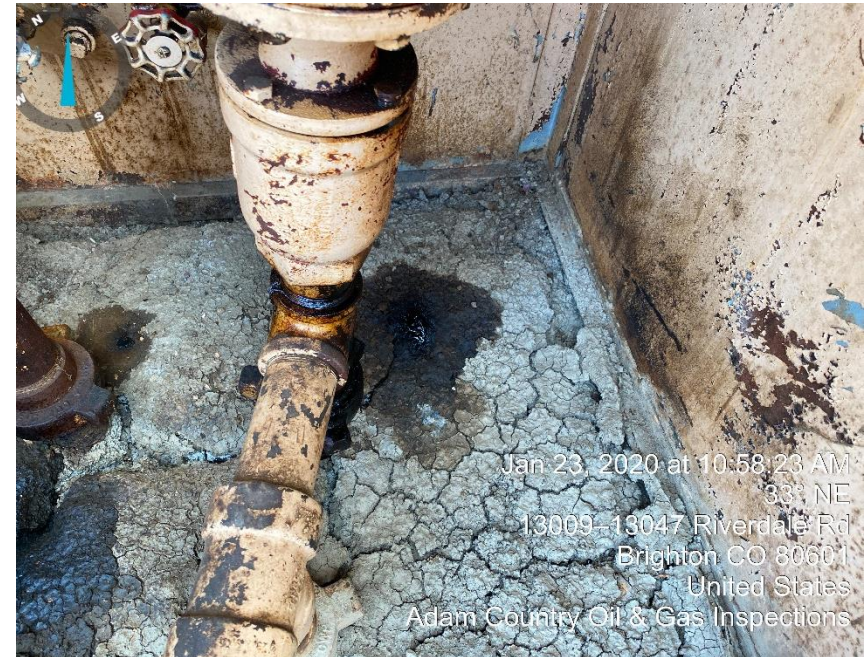
Photo #8 Stained soil under oil dump
