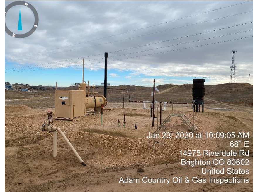
Photo#2 Separator, Combustor and Meter run
