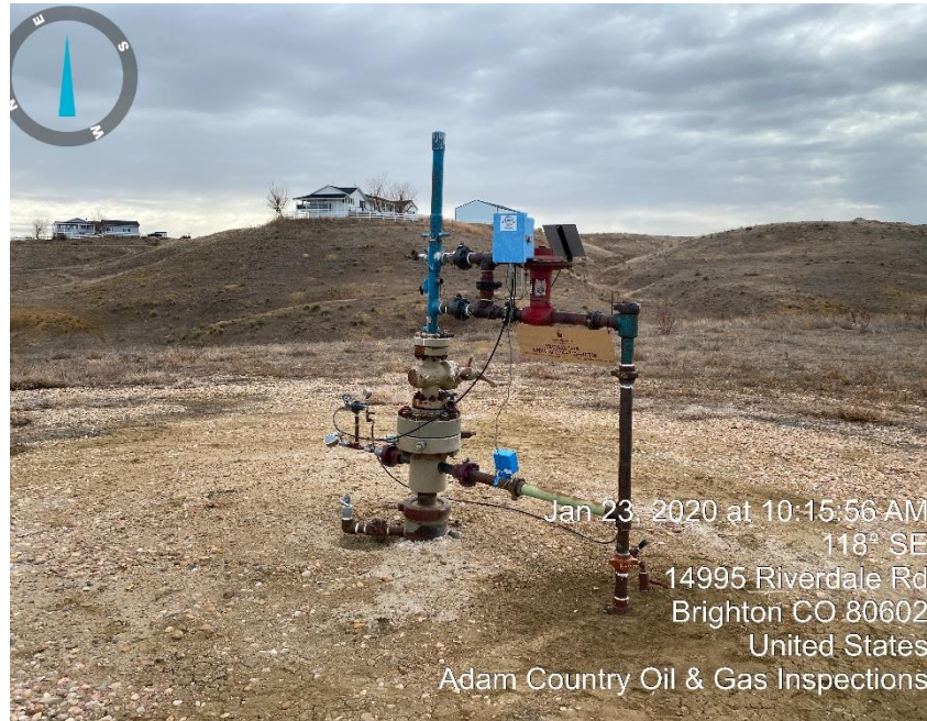
Photo #3 Well head
