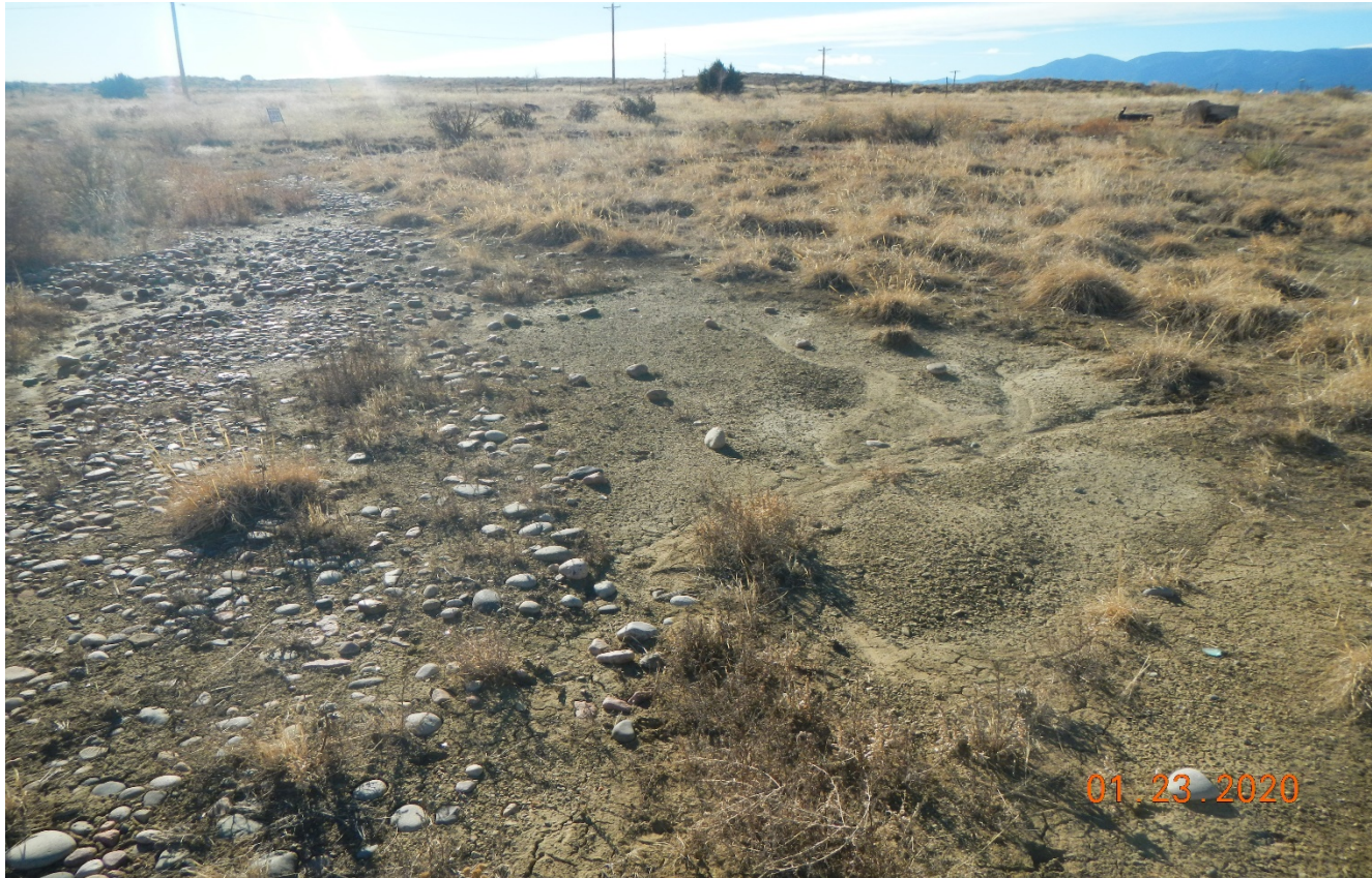
Photo 6. The access road made a circle around the well site. There is still gravel that remains and areas bare of vegetation along the former access road.
