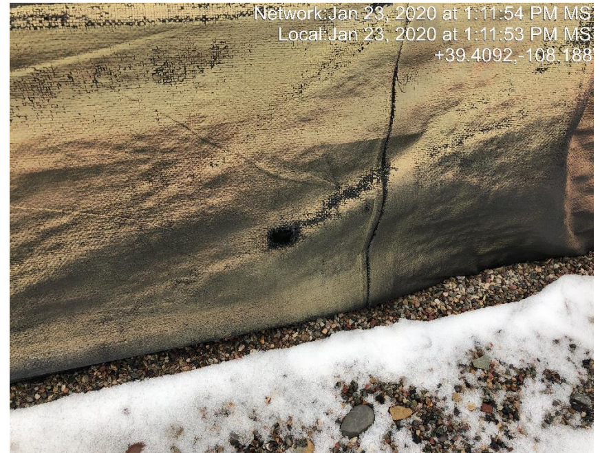
Photo #0455 Multiple holes in tank containment liner.
