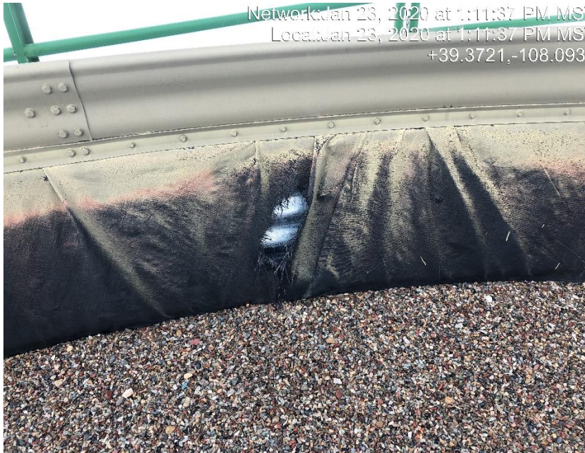
Photo #0454 Multiple holes in tank containment liner.
