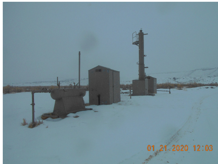
Separator, Meter housings and Dehydrator
