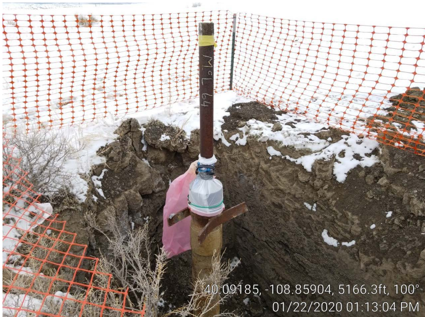
Photo 2. Bag attached to collect any gas leaking.
