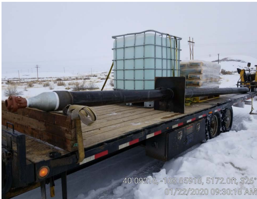
Photo 5. Surface casing installed 1-22-2020 to plug well.
