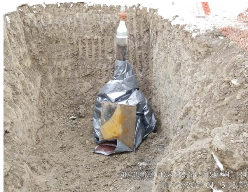
Photo 6. New surface casing installed.
