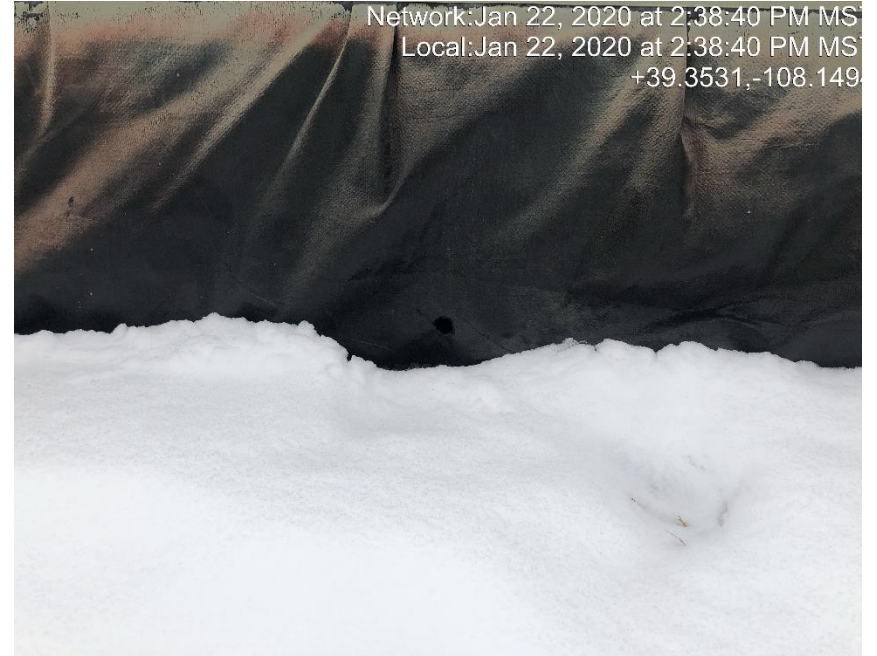
Photo #0446 Not all holes patched in tank containment liner.
