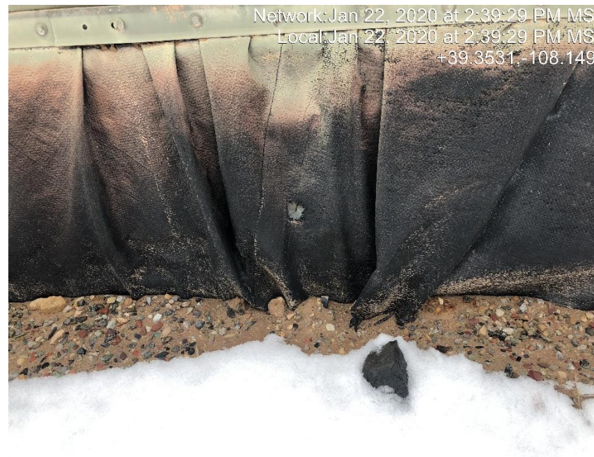
Photo #0448 Not all holes patched in tank containment liner.
