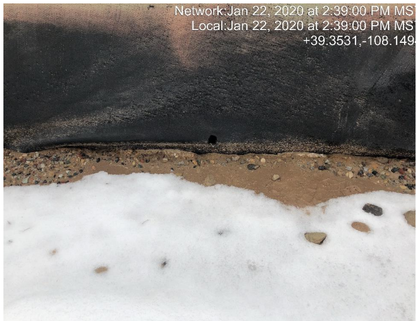
Photo #0447 Not all holes patched in tank containment liner.
